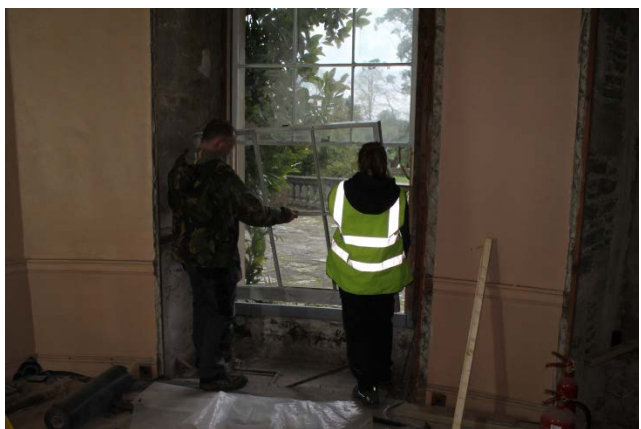
SARAH HUDSON REINSTATING A REPAIRED SASH WINDOW AT MOUNT STEWART HOUSE, NORTHERN IRELAND
