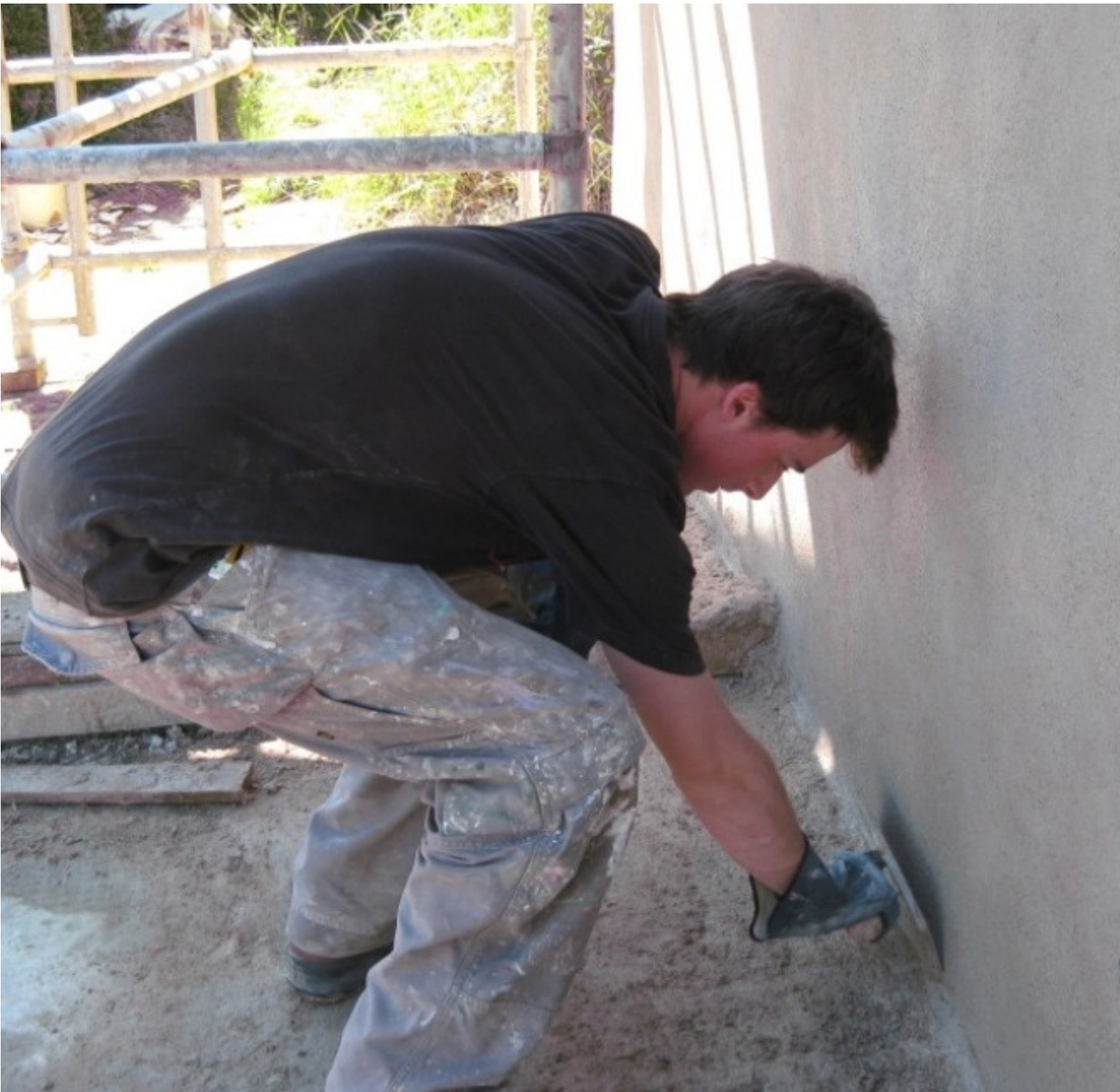
NED FLOYD APPRENTICE PLASTERER
