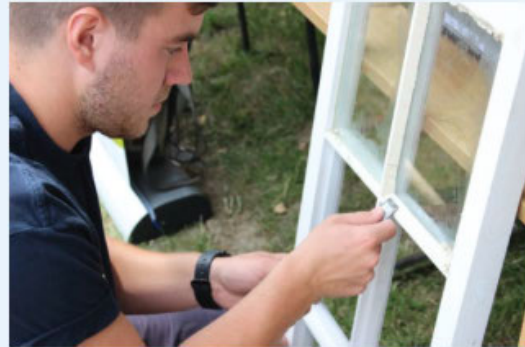
Trainee bench joiner Luke McEnroe working on traditional windows at the National Trust's Buscot and Coleshill estate. © National Trust TBSBS.
