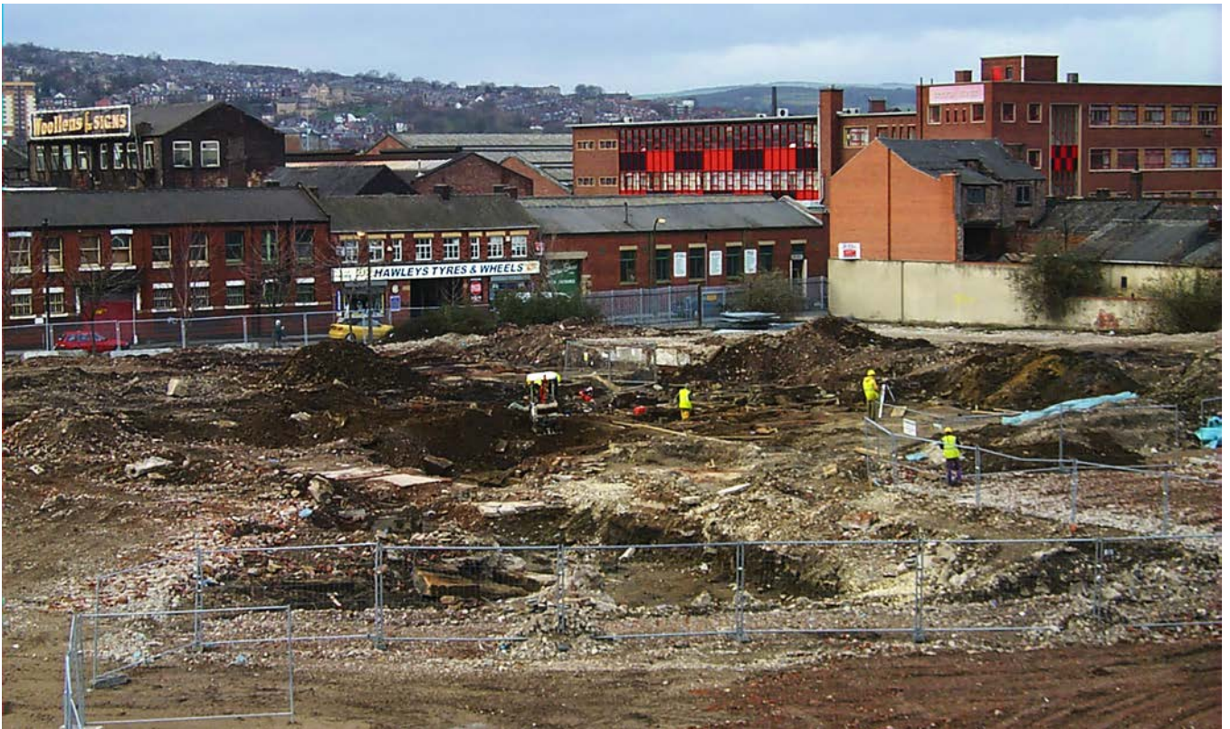
Figure 1 Early stages of the excavation on the Riverside Exchange site in central Sheffield. The scale of many sites of historic industries can be daunting.
