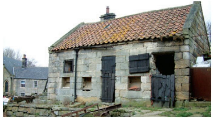
A pigsty in the North York Moors, with feeding chutes. Photo © Jen Deadman
