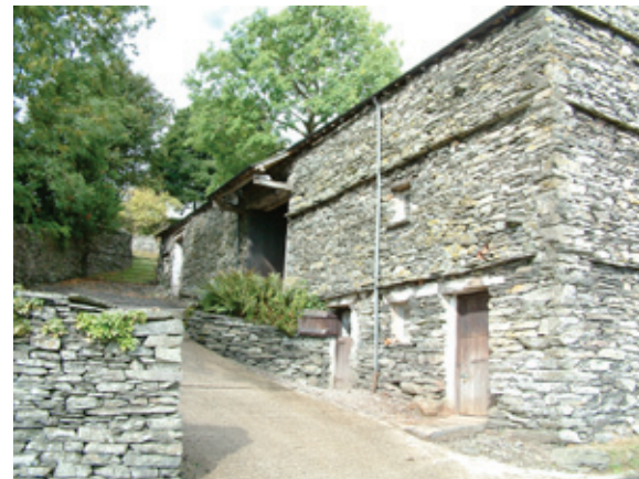
Variant bank barn in the Lake District, with a stable and cowhouse set in the downslope end and a small window marking a first-floor granary. Photo © Jen Deadman
