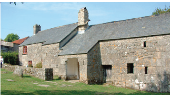
Sanders in Lettaford is one of the best-preserved longhouses in Dartmoor, now in the care of the Landmark Trust. It was built in the early 16th century, with the shippon to the right of the porch. The lean-to porch with its shouldered arch is probably original. Parallel to its north is a range comprising a late 18th-early 19th century barn, stable, cartshed and pigsties. Photo © Jeremy Lake
