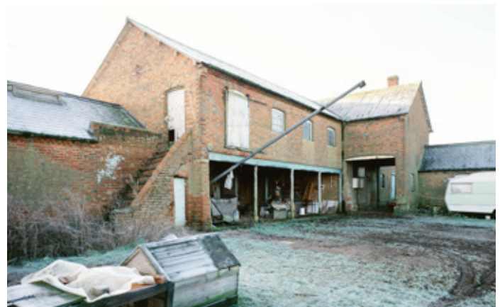
A large combination barn on the Duke of Bedford estate in Bedfordshire, typical of those on the largest courtyard plan farmsteads. It includes a granary sited above a large cartshed in the foreground and a projecting engine house, in which a portable engine would be parked and connected to internal gearing and machinery. Photo © English Heritage/ Mike Williams
