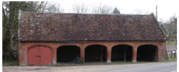
A four-bay cartshed with an additional implement shed, marked by lockable doors, on a large corn-producing farm in the Hampshire Downs. Photo © Bob Edwards
