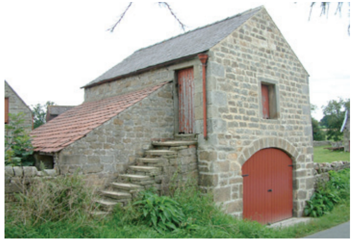
Single-bay cartsheds, as here in the Yorkshire Dales with steps to a first-floor granary, are typical of upland farms. Photo © Jeremy Lake
