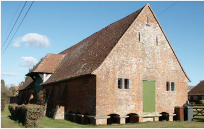
Some of the largest aisled barns in the arable vales and downs of southern England were built with integral stables and granaries, as here in this Hampshire Downs example, where the granary is raised on staddle stones. Photo © Bob Edwards
