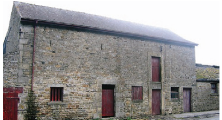
Storeyed barn from Weardale, Durham, showing a winnowing and loading door above a cow house and stables. This type of storeyed combination barn was built in large numbers in the late 18th and 19th centuries, often replacing earlier generations of cruck-framed barns, and is widely found in the Pennines and the south west (especially in an area from around Exmoor to Cornwall). Photo © Jeremy Lake
