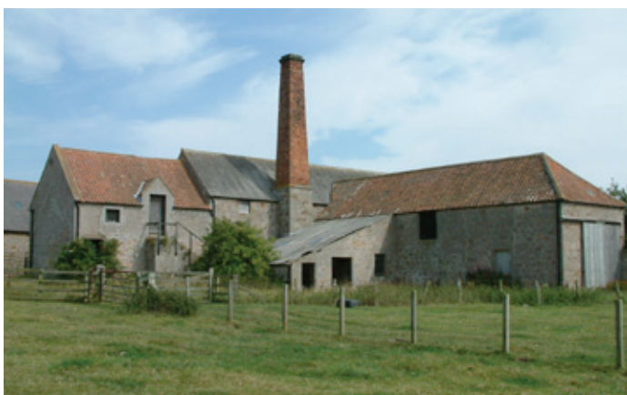
A chimneystack marks the position of a fixed steam engine in this planned farmstead in the Cheviot Fringe, Northumberland. To the left is a granary, marked by external steps, above a stable, and to the right is a projecting straw barn. Machine threshing produced large amounts of straw. Photo © Jen Deadman
