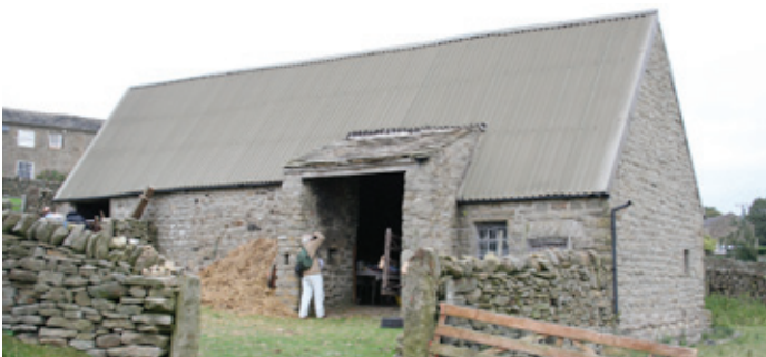
Cruck-framed barns are widely documented across the upland and upland fringe areas of northern England. They often had one end partitioned off for a cowhouse. The external walls on this example at Drebley in Wharfedale, Yorkshire Dales, are 18th century or possibly earlier, and replaced the original timber and wattle walls. Fragments of heather thatch survive inside. To the east downslope end of the barn is an external door to the former cowhouse, the cattle being tethered with their heads facing the stone-flagged threshing floor. To the west end of the barn is a root cellar; which is later 18th century or later in date. There are several root cellars with segmental-arched roofs in this area, which relate to the expansion in the cultivation of root crops and in particular potatoes. Photo © Jeremy Lake
