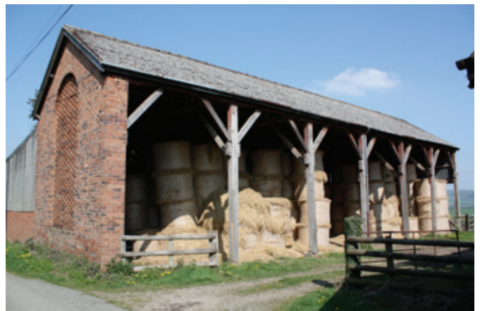
A mid-late 19th century hay barn on a planned farmstead built to house a large herd of dairy cattle, and the hay needed to feed them, in north Shropshire. Hay barns of this type, with brick piers or (as here) timber posts, are commonly associated with the large dairying farmsteads of this period found across the plains of Lancashire, Cheshire, Shropshire and Staffordshire. Photo © Jeremy Lake
