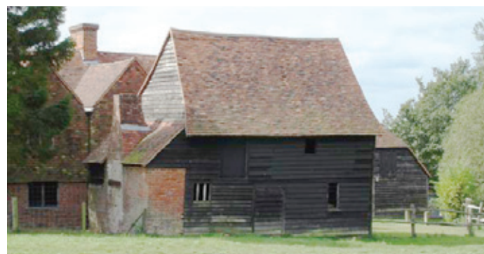
A rare survival of a detached kitchen to the rear of a High Weald farmhouse. Such buildings will often have smoke-blackened roof timbers to at least part of the roof and may have been partly floored. The stack at the gable end is a later addition. Photo © Steve Podd, FWAG
