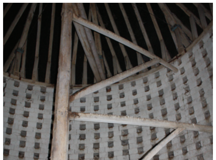
The interior of a mid 17th century dovecote in the Berkshire and Marlborough Downs showing the chalk block nesting boxes and the revolving ladder support, a rare survival. Photo © Bob Edwards
