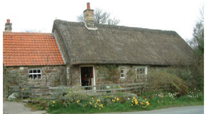
Former longhouse in the North York Moors, its lower end rebuilt as a service room entered off the through passage. Photo © Jeremy Lake
