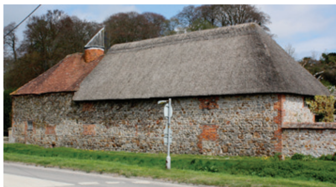
A rare example of a 19th century malthouse located on a village farmstead in the Marlborough Downs of Wiltshire that retains its characteristic cowled vent to the drying chamber. With the loss of this feature, it would be difficult to identify the function of this building without an internal inspection. Photo © Bob Edwards
