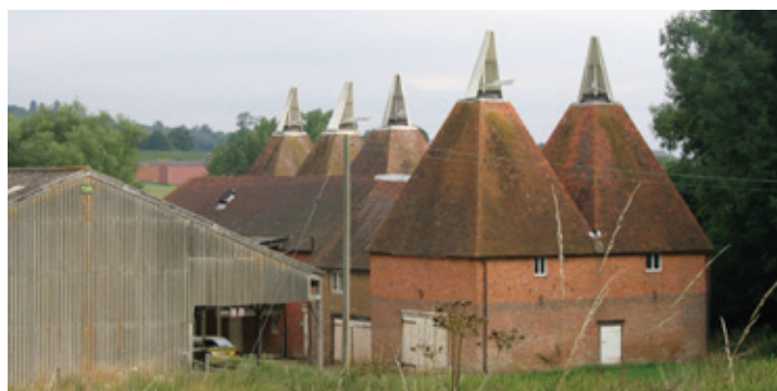
Square kilns, as here near Bromyard in Herefordshire, were introduced in the early 19th century. Photo © Jeremy Lake
