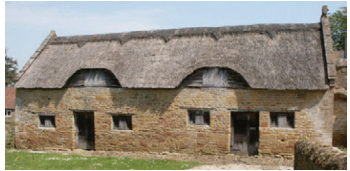
17th century stable at Stoke-sub-Hamdon in Somerset. Photo © Jeremy Lake
