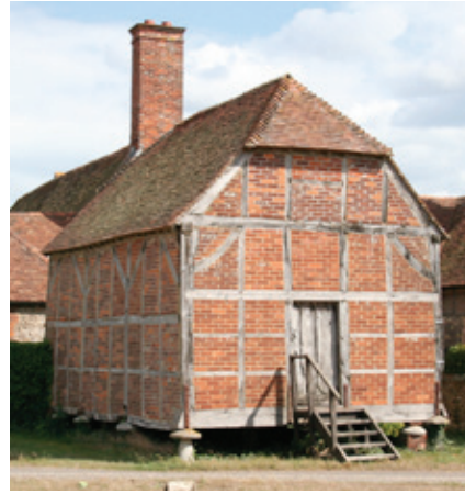
Detached 17th or early 18th century granary from south Hampshire built on staddle stones. Photo © Bob Edwards
