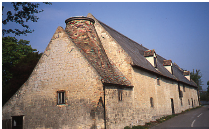
A malting in Cambridgeshire, showing the kiln in the foreground (East Anglian Chalk). Photo © Susanna Wade Martins
