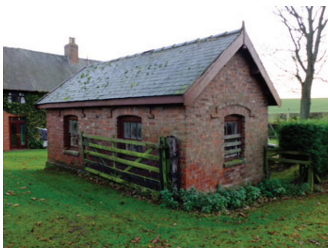
This slaughterhouse is part of a large late 19th century planned farmstead west of Hartlepool, its exterior revealing little of its original function. Photo © English Heritage
