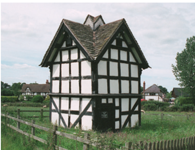
Seventeenth-century timber-framed dovecote in Herefordshire. Internally the nest boxes of this building are made from stone rubble, but wooden nest boxes and, in East Anglia, clay bats forming the nest boxes are also found. Photo © 149817 Mr Chris Tresise, taken as part of the Images of England project
