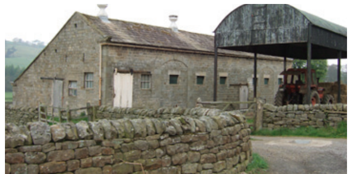
Late 19th century single-storey cow house, with ridge ventilators and detached hay barn, in Nidderdale. Photo © Jen Deadman
