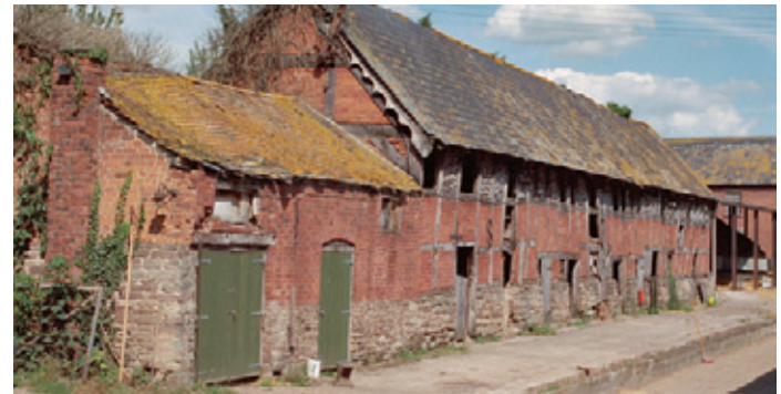
Two-storey timber-framed cow house in Herefordshire. Early cow houses of this type, with a first-floor hay loft, are found along and to the west of the Pennines, along the Welsh borders and in the south-west peninsula. Photo © Bob Edwards
