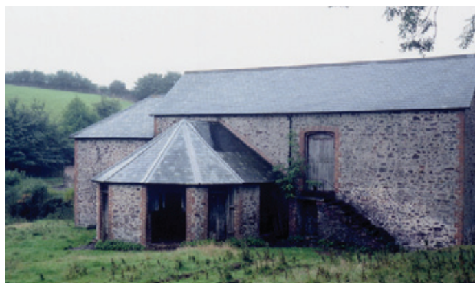
This horse-engine house forms an integral part of a bank barn in south Devon, typical of south-west and north-west England. Note the pitching door from the stack yard to the upper threshing area where the threshing machine was located, above the cattle housing. Photo © Jeremy Lake
