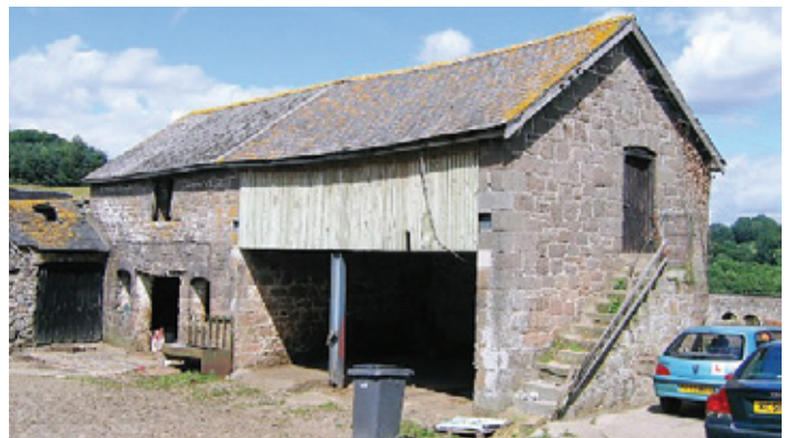
External steps mark the entrance to a granary sited above a 2-bay cartshed in the Oswestry Hills, attached to a stable. The whole range testifies to the intensification of arable farming in the mid 19th century in this upland area. Photo © Jeremy Lake
