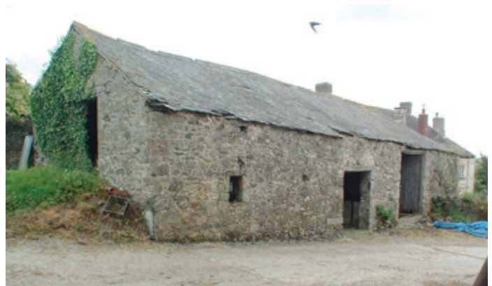
Cider barn to the east of Dartmoor; with a taking-in door accessed from the orchard to the left gable, a wide doorway to the cider mill and an open-fronted barrel store. Photo © Philip White
