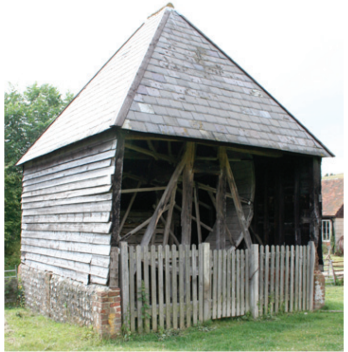
A very rare surviving example of a well house, in the South Downs, powered by a donkey wheel. Photo © Bob Edwards
