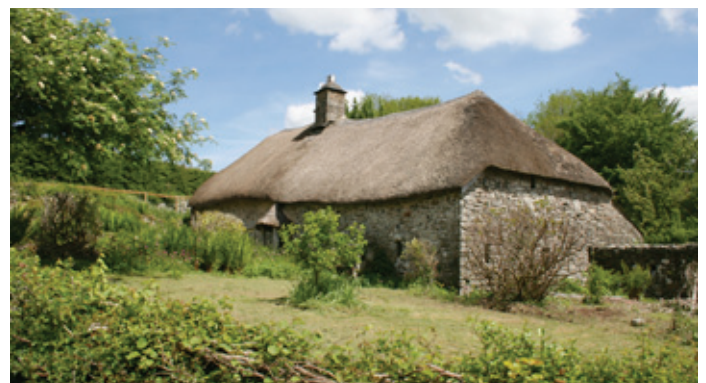
Higher Uppacott at Poundsgate is one of a group of four longhouses sited along the same lane in Dartmoor. The early 16th century house is built into the sloping ground, and the photograph shows the ventilation slits to the well-preserved lower shippon end which retains its central drain © Dartmoor National Park Authority
