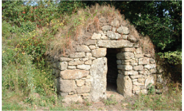
An example from the east of Dartmoor with a corbelled stone roof found associated with these buildings and also dovecotes and pigsties in south west Wales and north west France. Photo © Philip White
