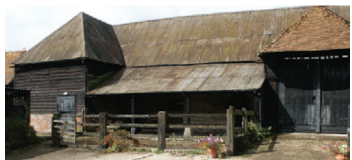
Shelter sheds, and other forms of cattle housing, can be found attached to earlier barns as here bordering the Hampshire Downs. Photo © Bob Edwards
