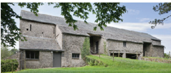
An early 19th century bank barn from east Cornwall, showing the access from the rear to the threshing floor above housing for cattle. © English Heritage
