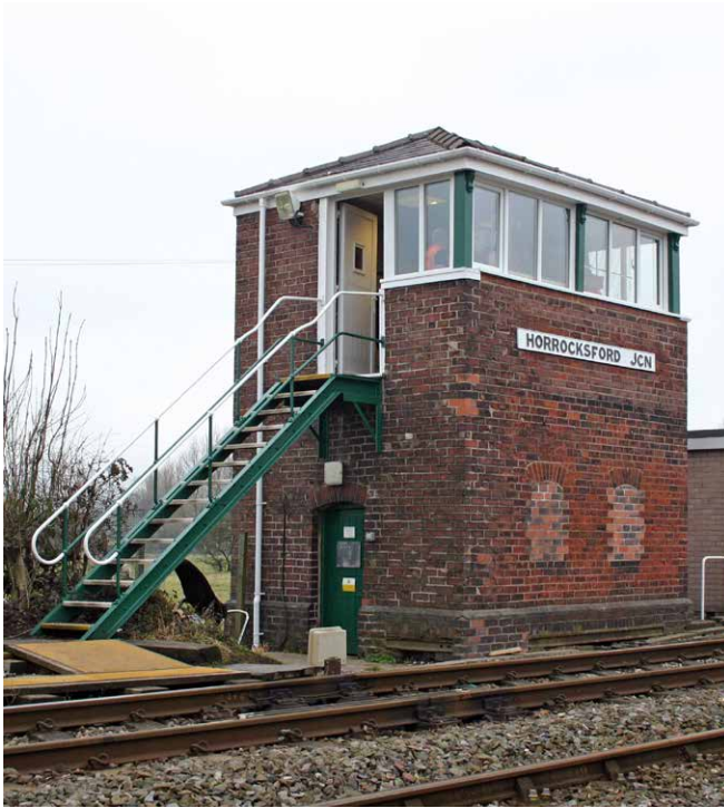
Figure 16 Early signal boxes tended to be quite plain in appearance, with little of the decoration found in many boxes of the 1880s. Horrocksford Junction (Lancashire;1873), is an example of the early Saxby & Farmer designs for northern companies, in this case the L&YR. It has undergone major alterations as part of the Railtrack/Network Rail modernisation programme, including replacement windows and steps and has had the locking room windows bricked up.
