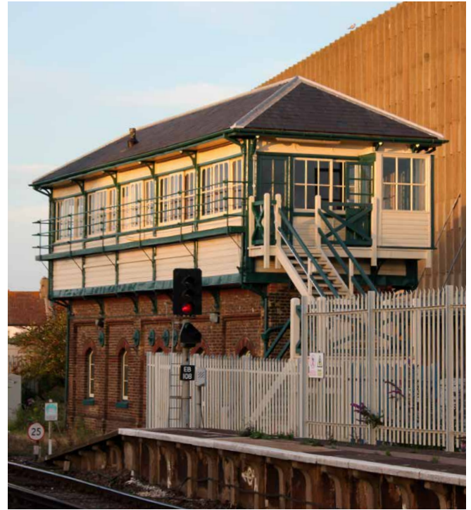
Figure 17 The Saxby & Farmer type 5, with shaped eaves brackets and round-cornered upper lights, is highly distinctive. Eastbourne's (East Sussex; 1882, listed Grade II) is one of the largest. Space was tight, and the timber superstructure is cantilevered from a narrow brick base enlivened by polychrome brickwork and pointed arches to the locking room windows. This echoes the elaboration of Eastbourne station.
