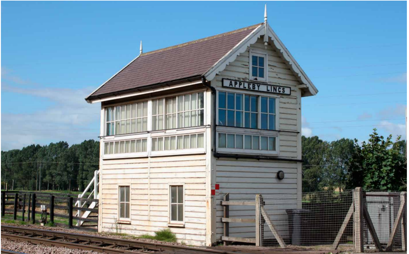
Figure 2 Appleby (Lincolnshire). A Railway Signal Co box (listed Grade II), built for the Manchester, Sheffield & Lincolnshire Railway (later GCR) in 1885. It displays the
