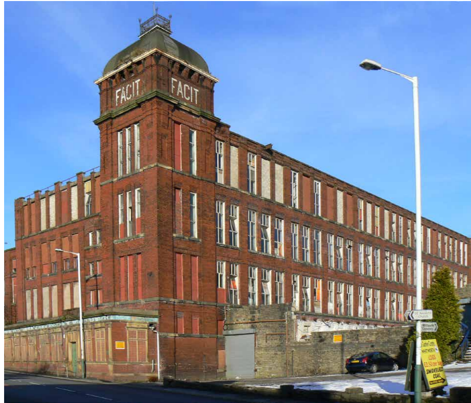
Left: Facit Ring Mill, near Whitworth in 2009, shortly before its demolition. © Oxford Archaeology Ltd
