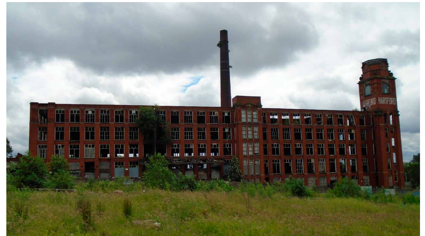
Above right: The derelict Hartford Mill in Oldham, a Grade II listed building beyond economic repair after being subject to a series of fires and vandalism. © University of Salford
