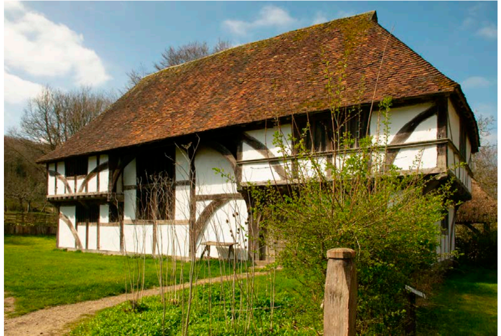
Figure 4: Bayleaf Farmhouse, a timber-framed Wealden hall house originally from Chiddingstone in Kent, re-erected at the Weald and Downland Museum in Singleton, West Sussex. © Andy Bliss
