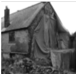
SITE NAME: Pridhamsleigh Farmhouse, Ashburton, Staverton
