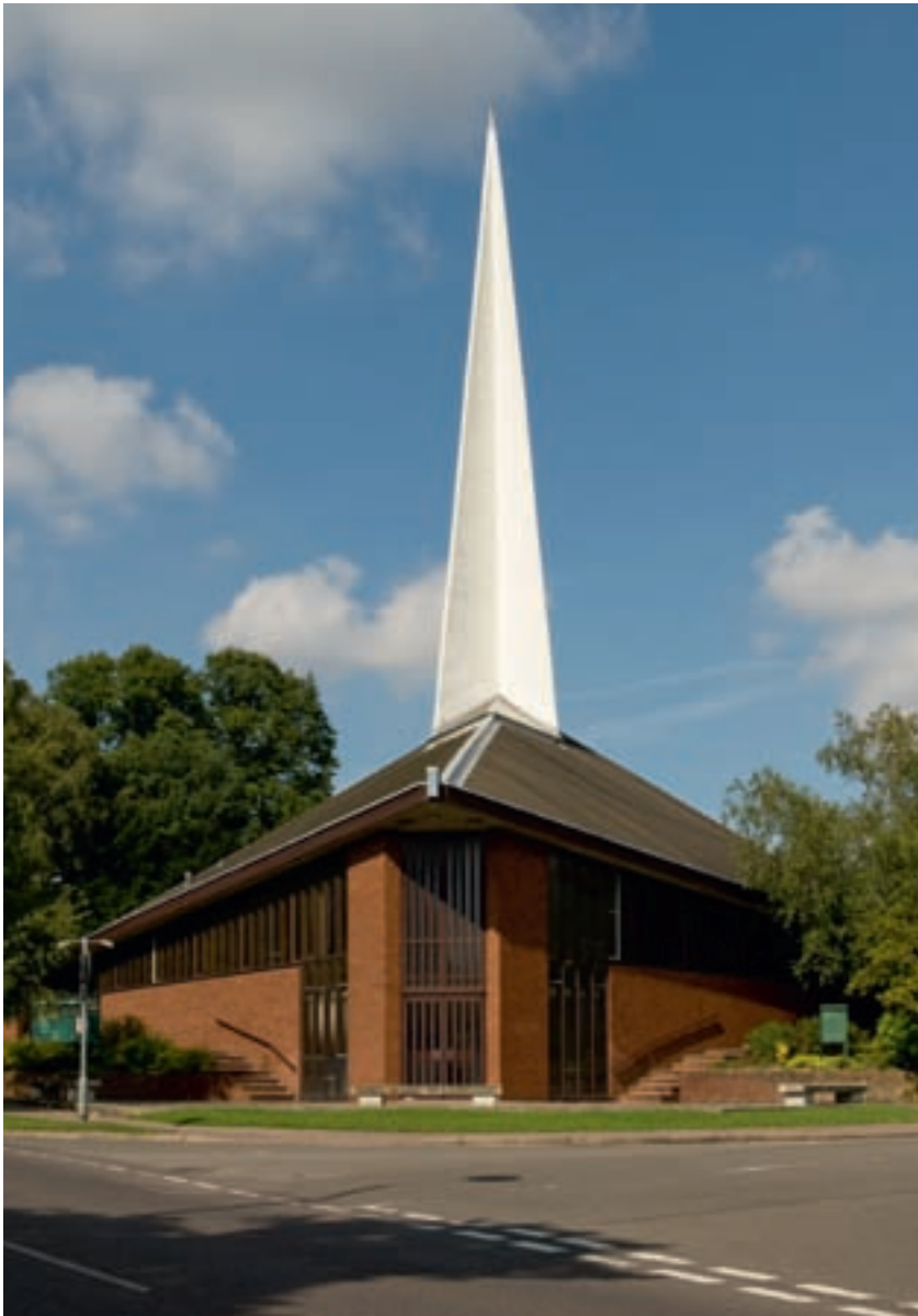
Figure 85 St George's, Norton Way North, Letchworth, with its landmark concrete flèche, 1964, by Peter Bosanquet of Brett, Boyd and Bosanquet. [DP088213]
