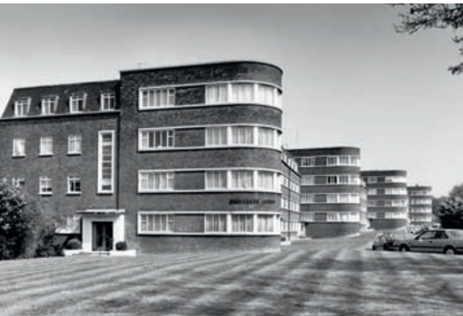
Figure 62 Belvedere Court flats, Lyttelton Road, designed by Ernst Freud in 1935, with bold 'streamform' bays. [Hampstead Garden Suburb Trust (Jane Whitton)]
