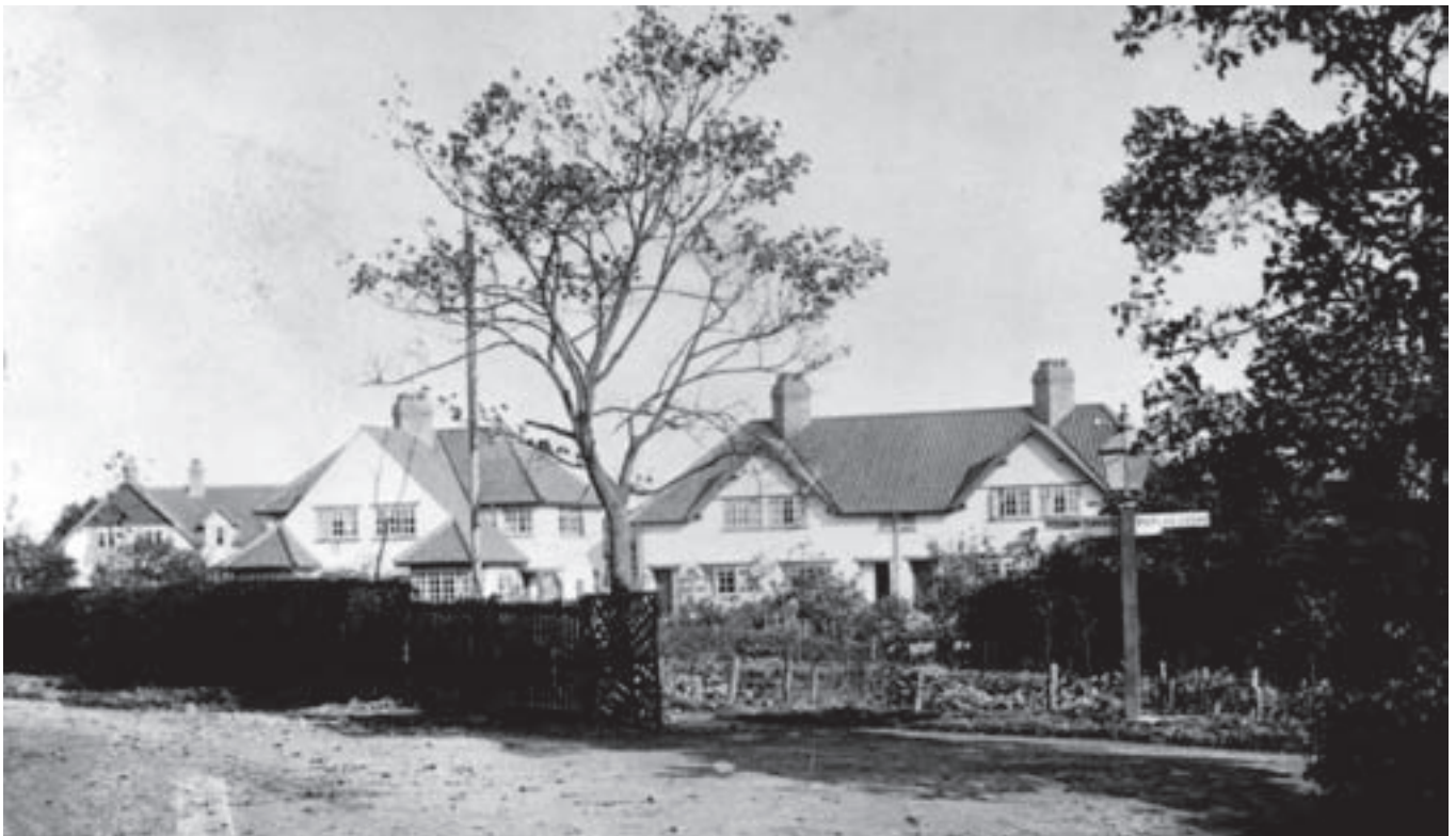
Figure 12 Western Terrace, New Earswick, 1902–3: group cottage prototypes for Letchworth. [© First Garden City Heritage Museum]
