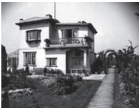
Figure 32 No 158 Wilbury Road: 1905 exhibit designed by John Alexander Brodie, city engineer of Liverpool, in a radical heavy concrete panel system. [© First Garden City Heritage Museum]
