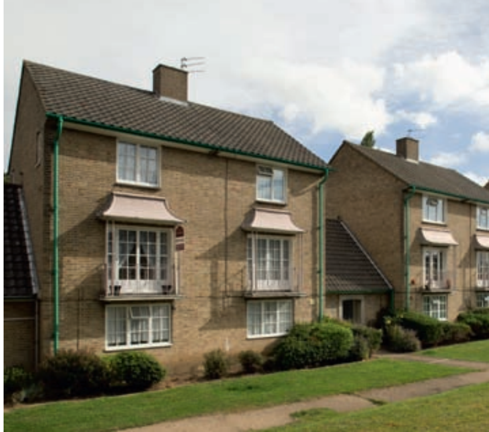
Figure 96 Knightsfield Flats, Welwyn Garden City, for New Town Development Corporation, 1955, by Louis de Soissons. [DP088302]
