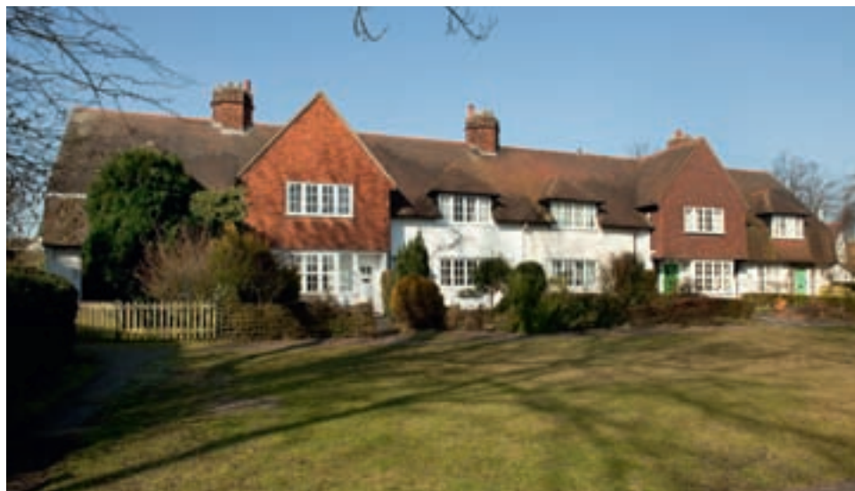
Figure 33 Nos 7–17 (odd) Lytton Avenue (originally Middle Street): prizewinning cottages designed by Courtenay Melville Crickmer for the 1907 Urban Cottages Exhibition. [DP088436]
