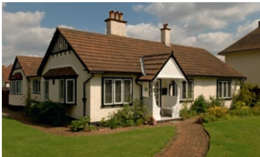
Figure 31 'The Nook', No 2 Cross Street: 1905 exhibit designed by Clare and Ross, now sensitively restored and extended. [DP088212]
