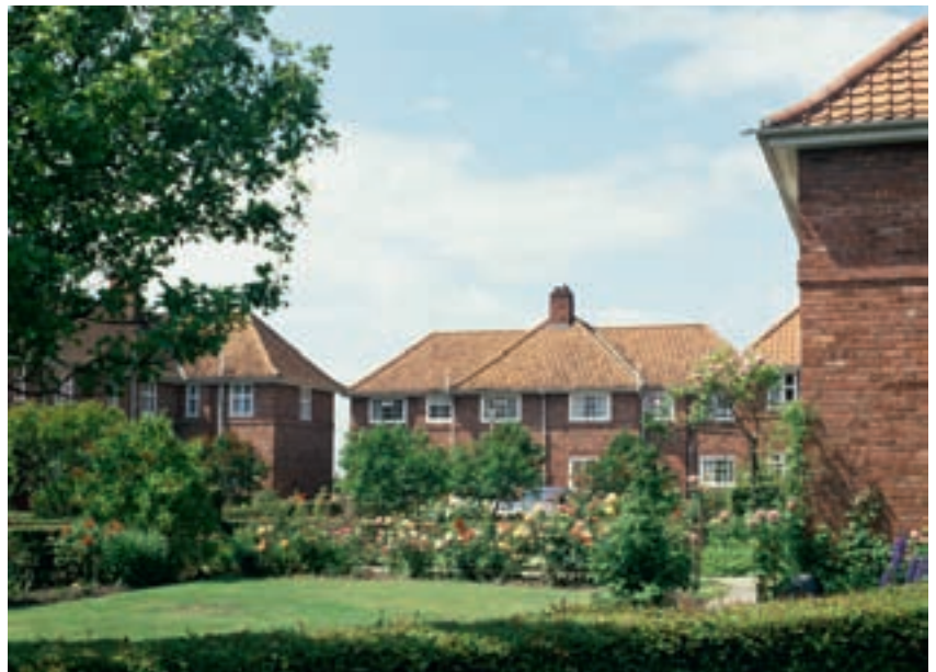
Figure 91 Barry Parker's cul-de-sac groupings at Wythenshawe were influenced by his contemporary inter-war work at New Earswick. [Mervyn Miller]
