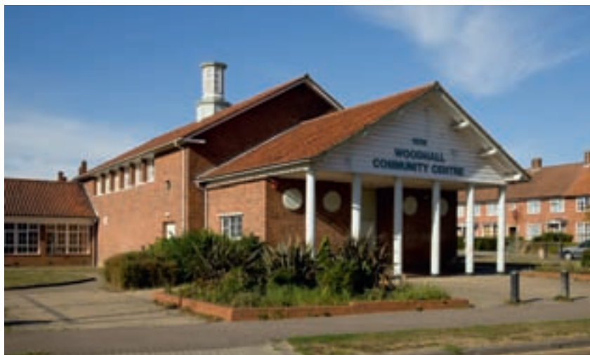
Figure 60 Woodhall Community Centre, Welwyn Garden City, 1938, by Louis de Soissons. [DP088309]
