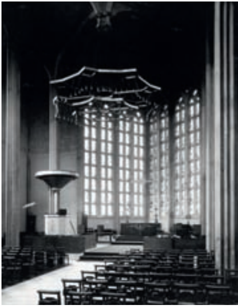
Figure 93 (above) The remarkable concrete Deco-Gothic interior of St Michael's and All Angels, Northenden, Wythenshawe, 1935–7, designed by Cachemaille-Day and Lander. [Manchester Archives and Local Studies, Central Library]
