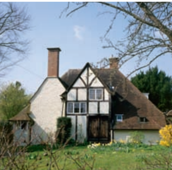
Figure 48 No 29 Norton Way North: of six Letchworth houses by M H Baillie Scott, this remains the least altered. [Mervyn Miller]
