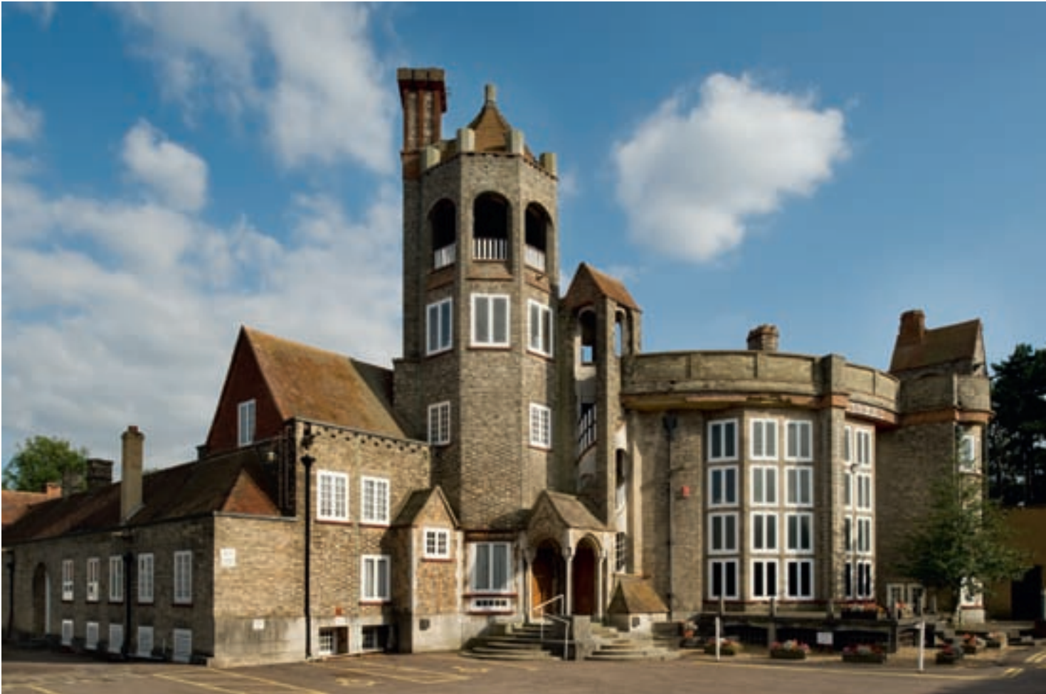
Figure 82 The Cloisters, Barrington Road, Letchworth, 1906–7, by W H Cowlshaw for Annie Jane Lawrence is now the North Hertfordshire Masonic Centre. [DP088242]
