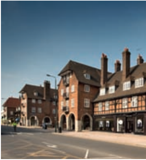
Figure 24 The Hampstead Way gateway group at Temple Fortune, 1909–11, viewed from Finchley Road was designed by Arthur Joseph Penty in Raymond Unwin's office. [DP110937]
