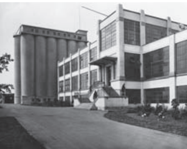
Figure 68 (above) The Shredded Wheat Factory and grain silo: a landmark of Welwyn Garden City, designed in 1924–5 by Louis de Soissons. [Hertfordshire Archives and Local Studies]
