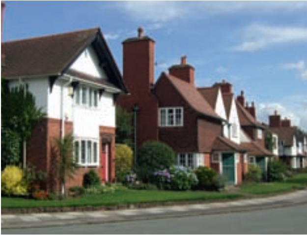
Figure 5 (above) Corniche Road, Port Sunlight. The cottages in the middle distance were designed by Edwin Lutyens in 1897. [Mervyn Miller]
