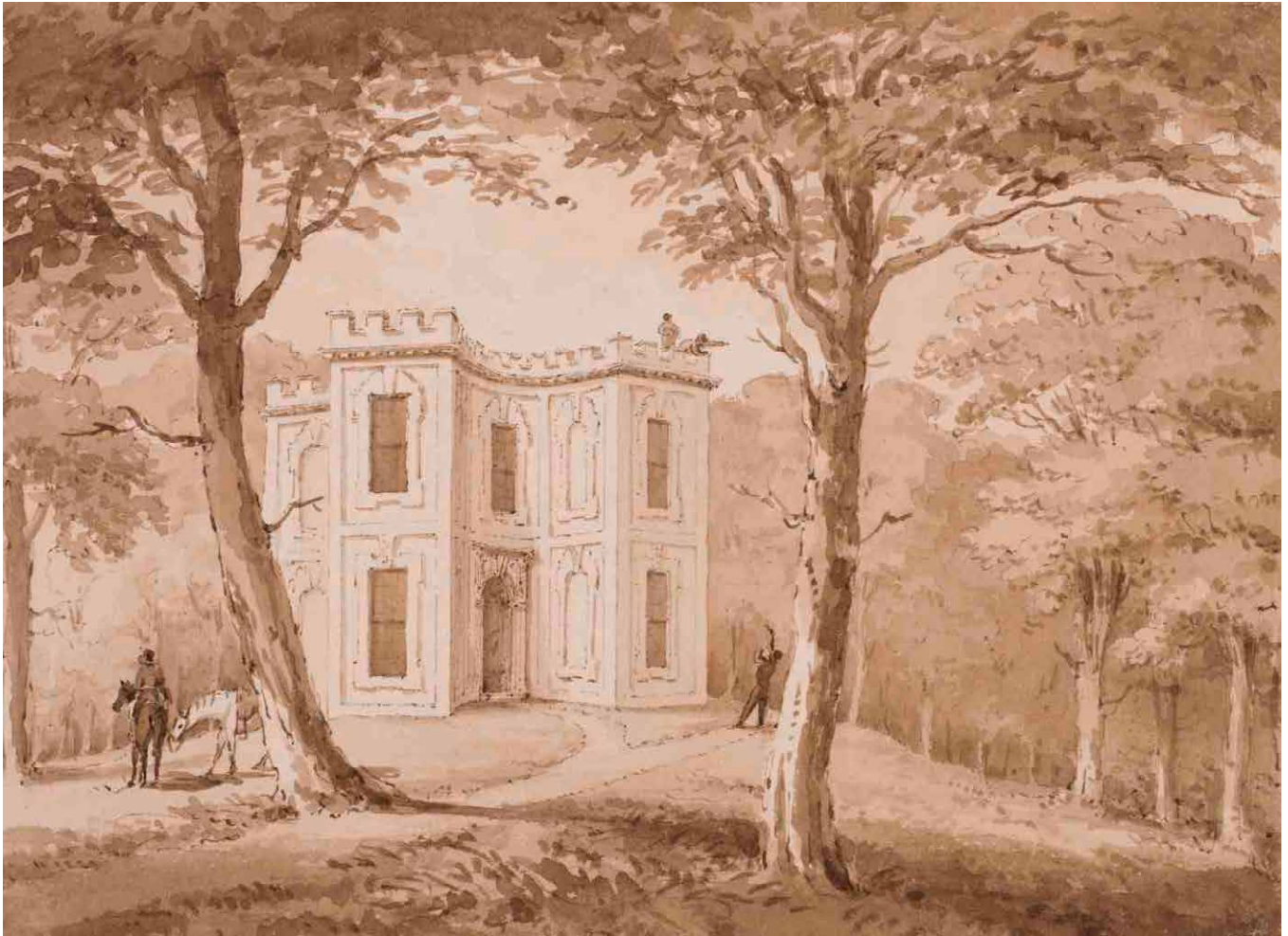
Figure 9 Cain Hill House, Wrest Park, Bedfordshire. Thomas Archer's garden building of about 1715 was a key element in this major designed landscape, included
