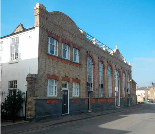
Figure 11 Crompton's Arc works, Anchor Street, Chelmsford, Essex. A simple utilitarian building designed, in imitation of an orangery, to house electrical generating plant and offices for R E B Crompton in 1878. Chelmsford had the first electric street lighting in the country, supplied by the Arc Works, in 1901. Listed Grade II.
