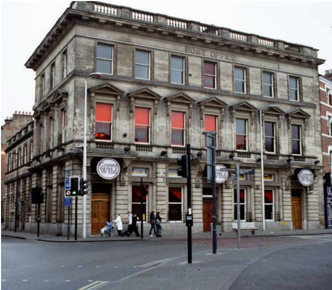
Figure 14 General Post Office, Victoria Street, Derby, Derbyshire. An early (1868) purpose-built head Post Office based on Renaissance precedents and resembling a London gentleman's club more than a new nineteenth-century building type. Listed Grade II.
