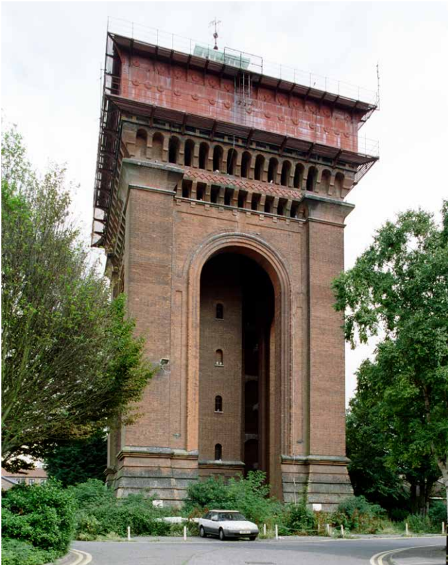
Figure 8 Municipal Water Tower, Balkerne Passage, Colchester, Essex. Opened in 1883, alongside is an early nineteenth-century reservoir, this enormous campanile, nicknamed ‘Jumbo’, was designed by the Borough Surveyor and Engineer Charles Clegg. Listed Grade II*.
