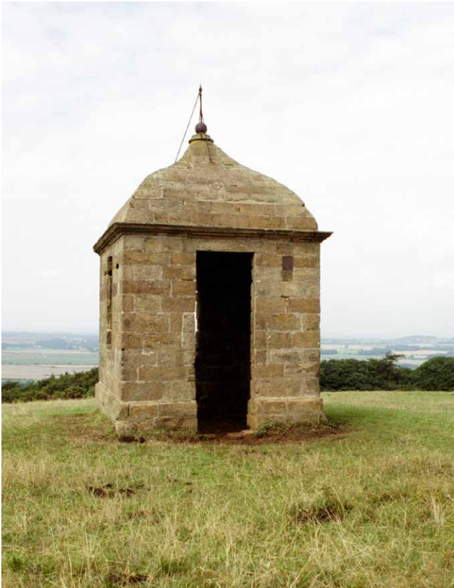
Figure 8 A shooting box of the late eighteenth century gave welcome rest, and cover, on this isolated spot in at Roseberry Topping in Great Ayton, North Yorkshire. Listed Grade II.
