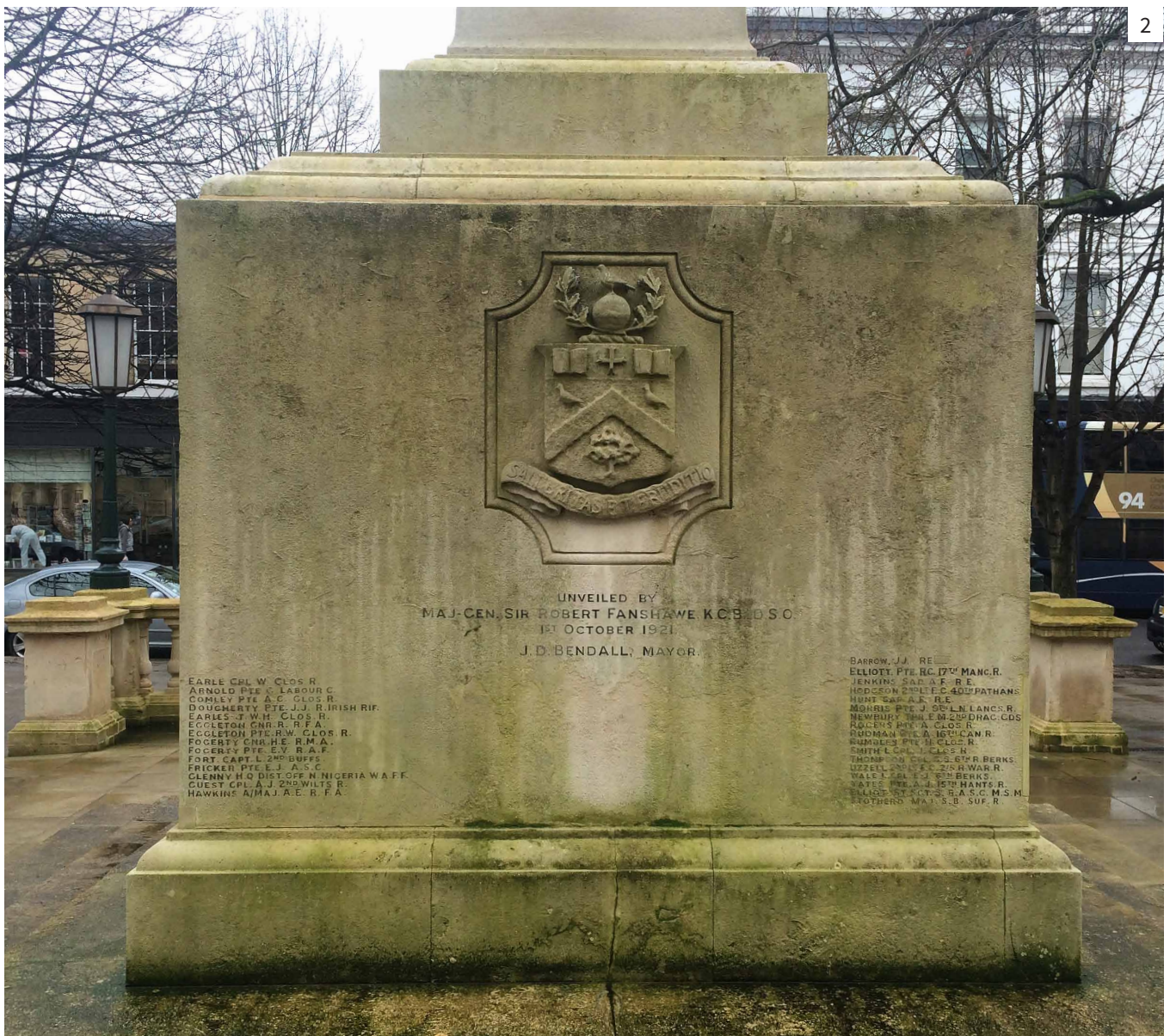
2 View of Cheltenham war memorial showing algal and lichen growth on west side.
