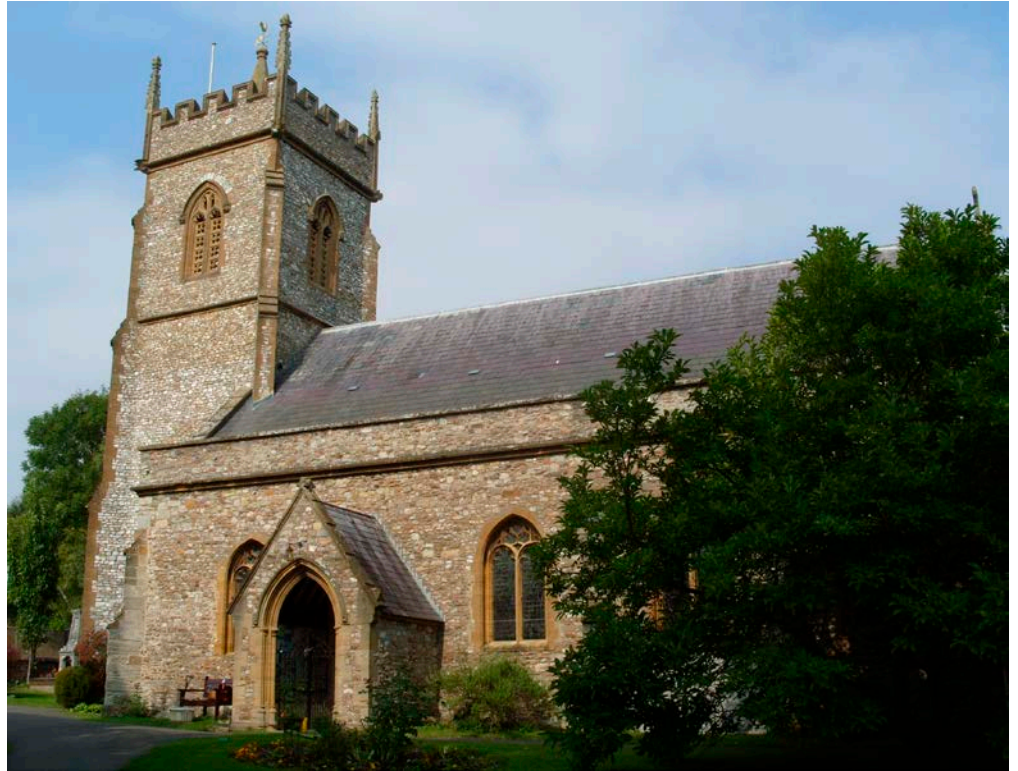
Figure 22: St George's Church, Wilton. Chert with Ham Hill Stone tracery, tower ornament and quoins.
