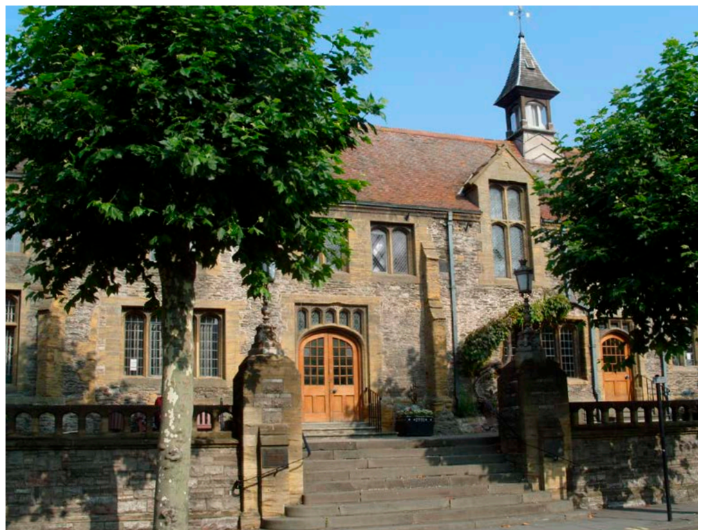
Figure 5: Old Municipal Buildings, Taunton. Morte Slates with Ham Hill Stone windows, dressings and buttresses.
