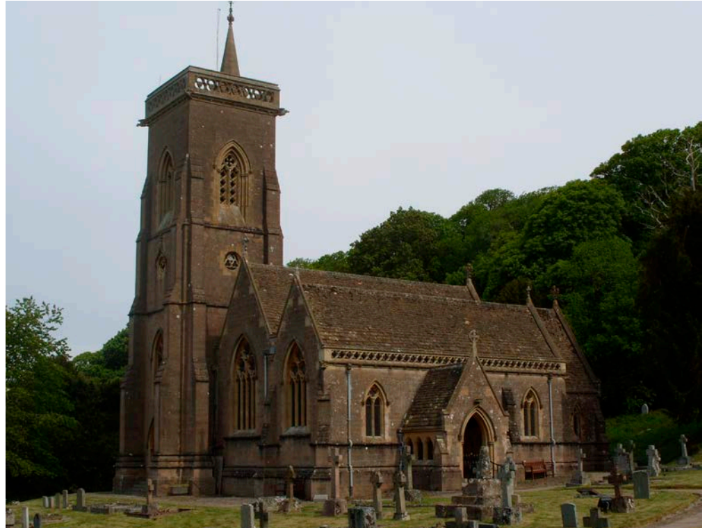
Figure 19: St Etheldreda's Church, West Quantoxhead. Douling Stone with Bath Stone dressings and tracery.
