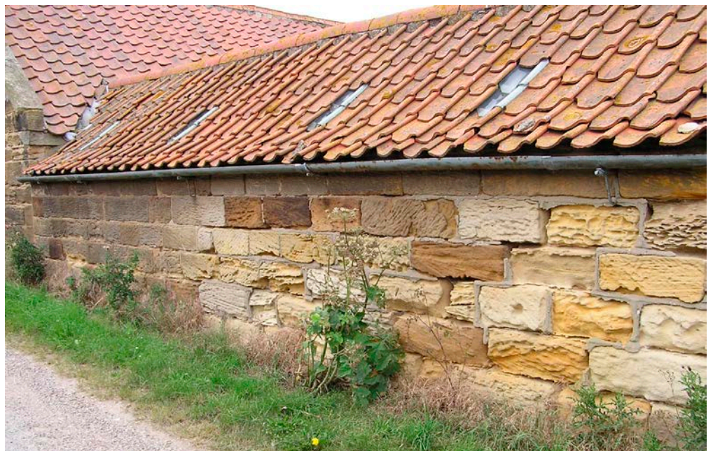
Figure 9: Farm building. Aislaby Stone.
