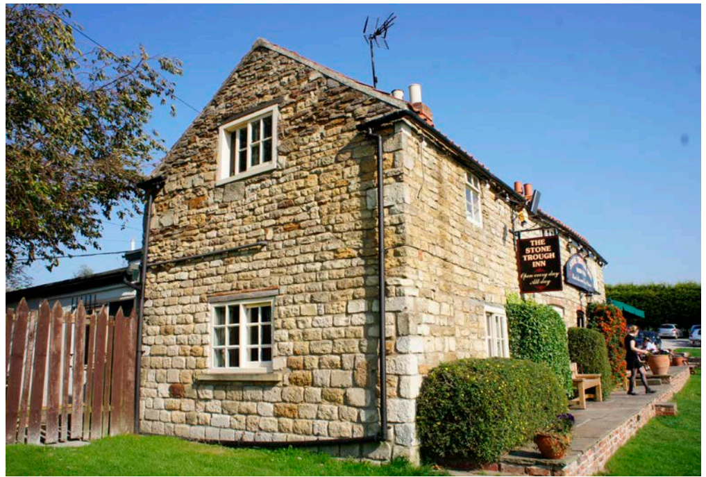
Figure 11: The Trough Inn, Kirkham. Whitwell Oolite and Dogger Formation Sandstone, and Corallian Group limestone quoins.
