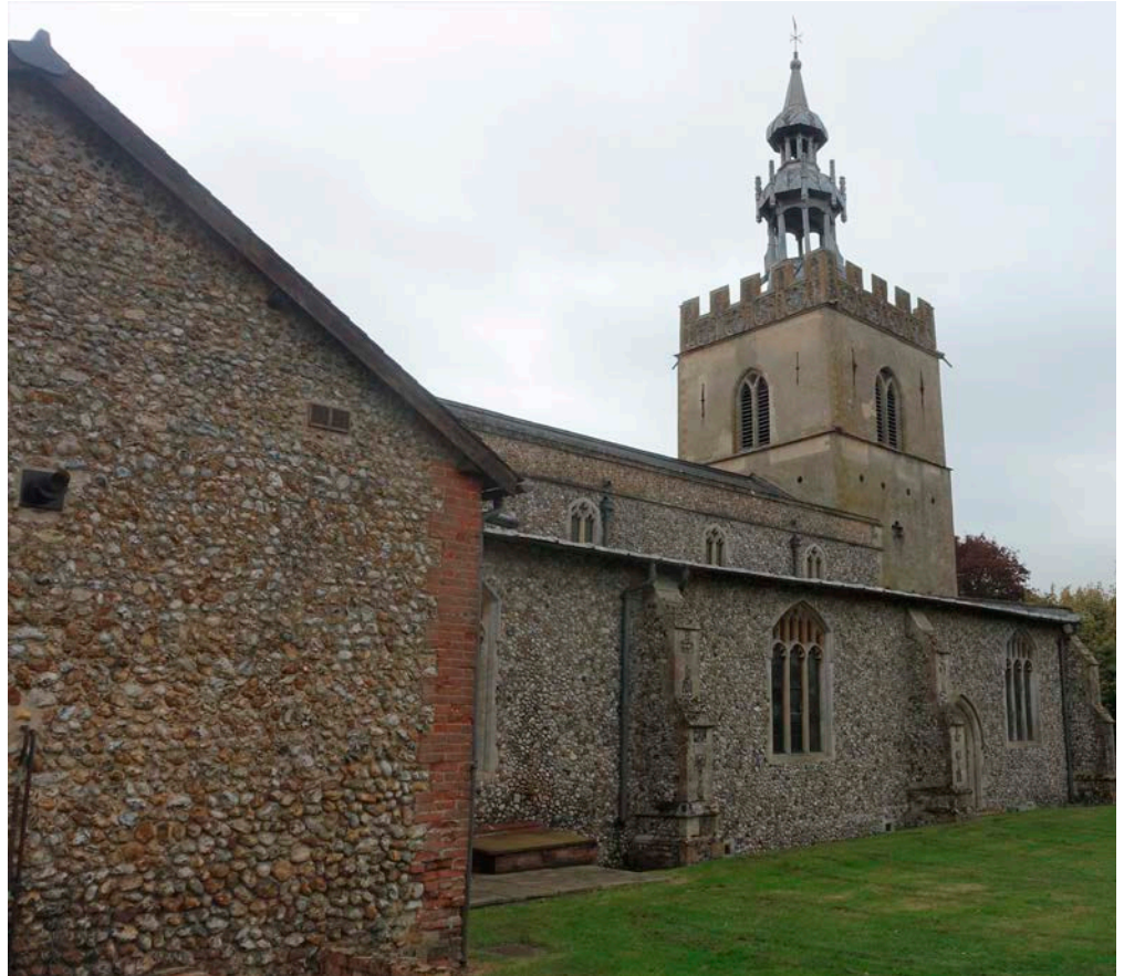
Figure 51: Church of All Saints, Shipdham. Chert pebbles and cobbles.
