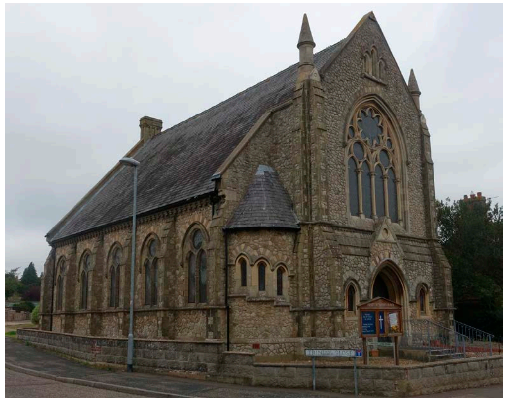
Figure 73: Trinity Methodist Church, Dereham. Kentish Ragstone with Bath Stone dressings.
