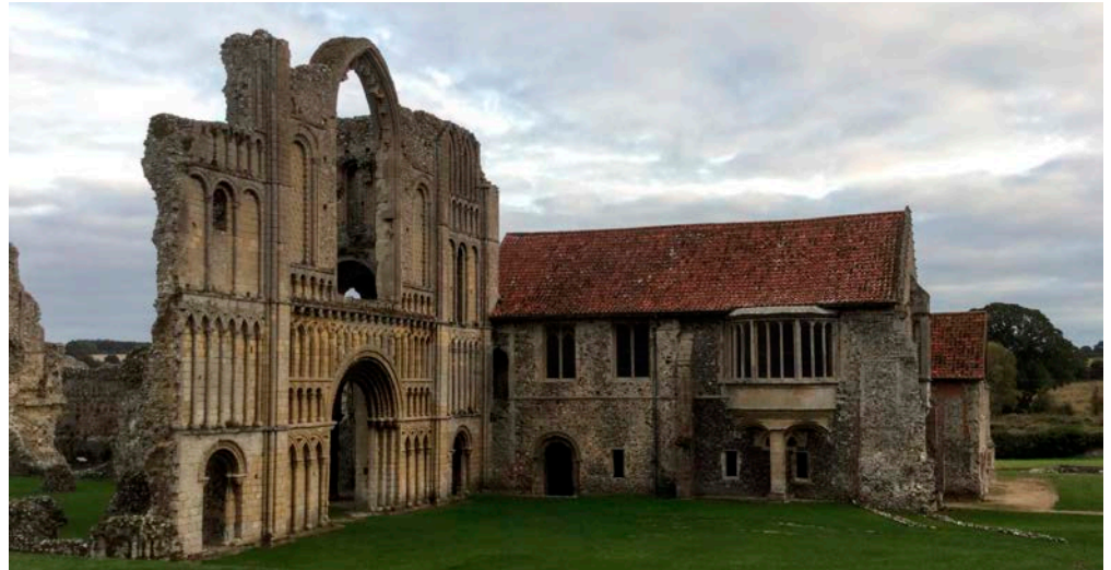
Figure 2: Priory and parlatorium, Castle Acre. Flint rubble with some chalk and carstone and Lincolnshire Limestone dressings.
