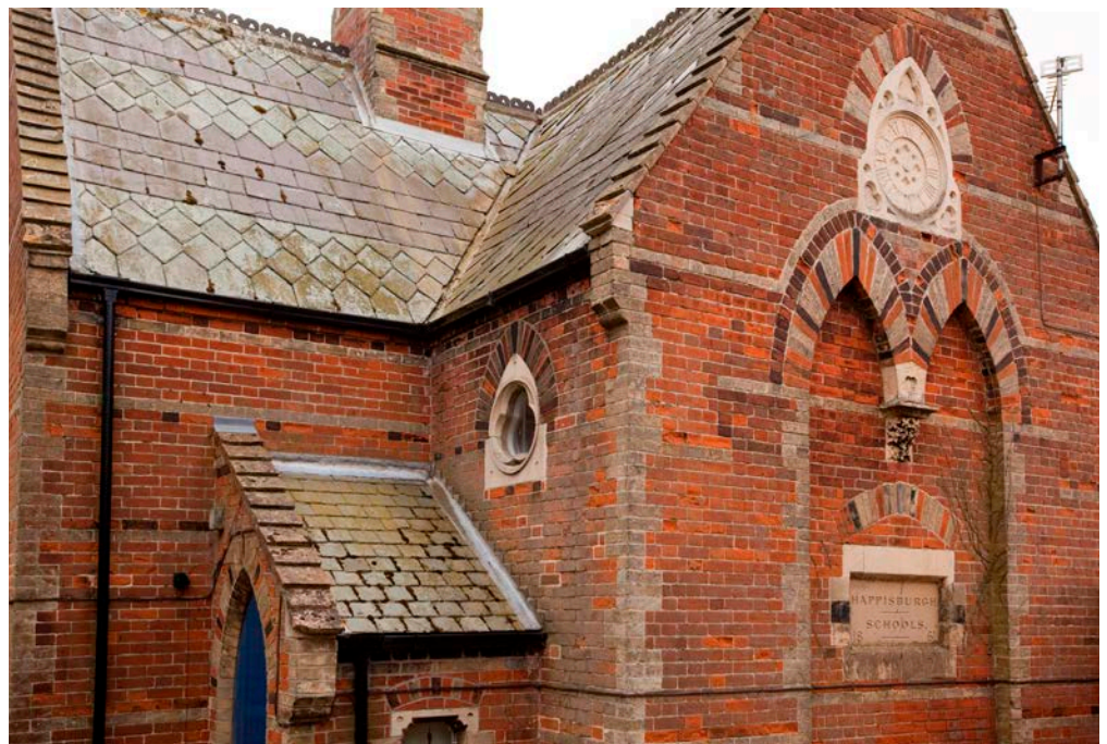
Figure 77: School, Happisburgh. Welsh Slate and (possibly) Westmorland Slate roof.
