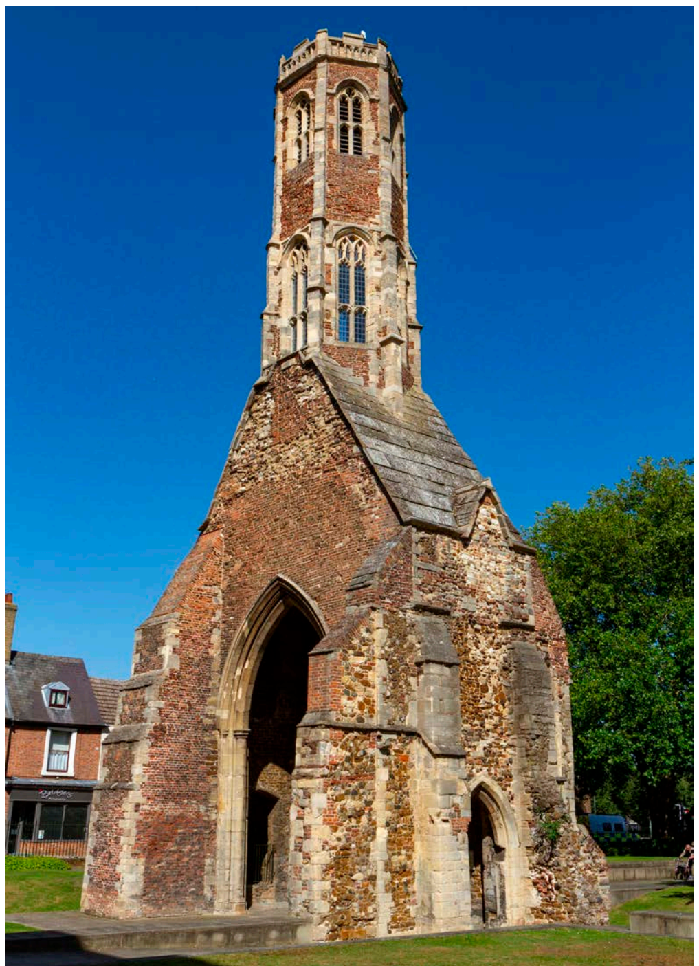
Figure 8: Greyfriars, King's Lynn. Carstone facing with Lincolnshire Limestone dressings.
