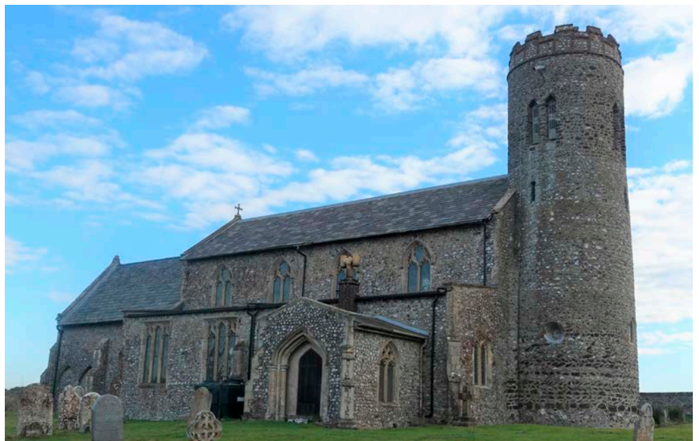
Figure 55: Church of St Mary, Roughton. Quaternary Flint and ironbound conglomerate.
