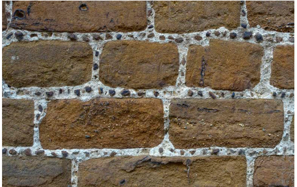
Figure 33: Tabular blocks of Big Carr with galletting.
