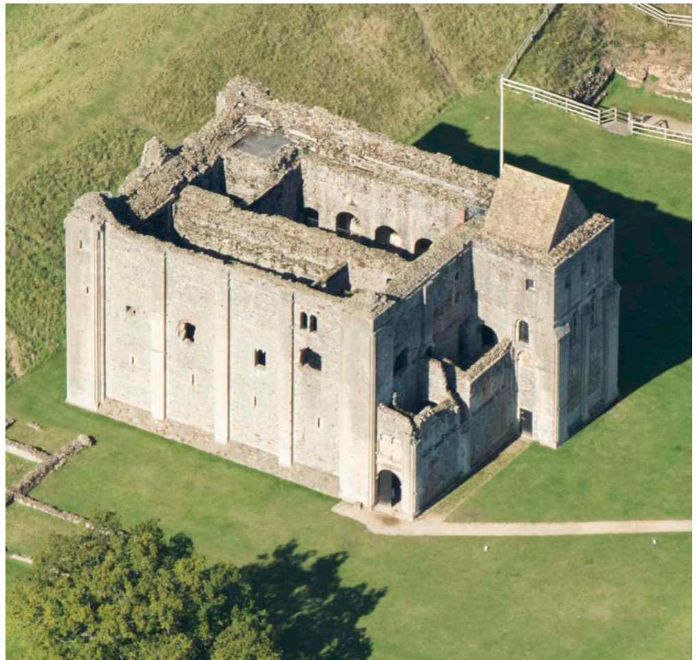
Figure 1: Stone Keep, Castle Rising. Lleziate Quartzite with Lincolnshire Limestone pilasters and quoins.
