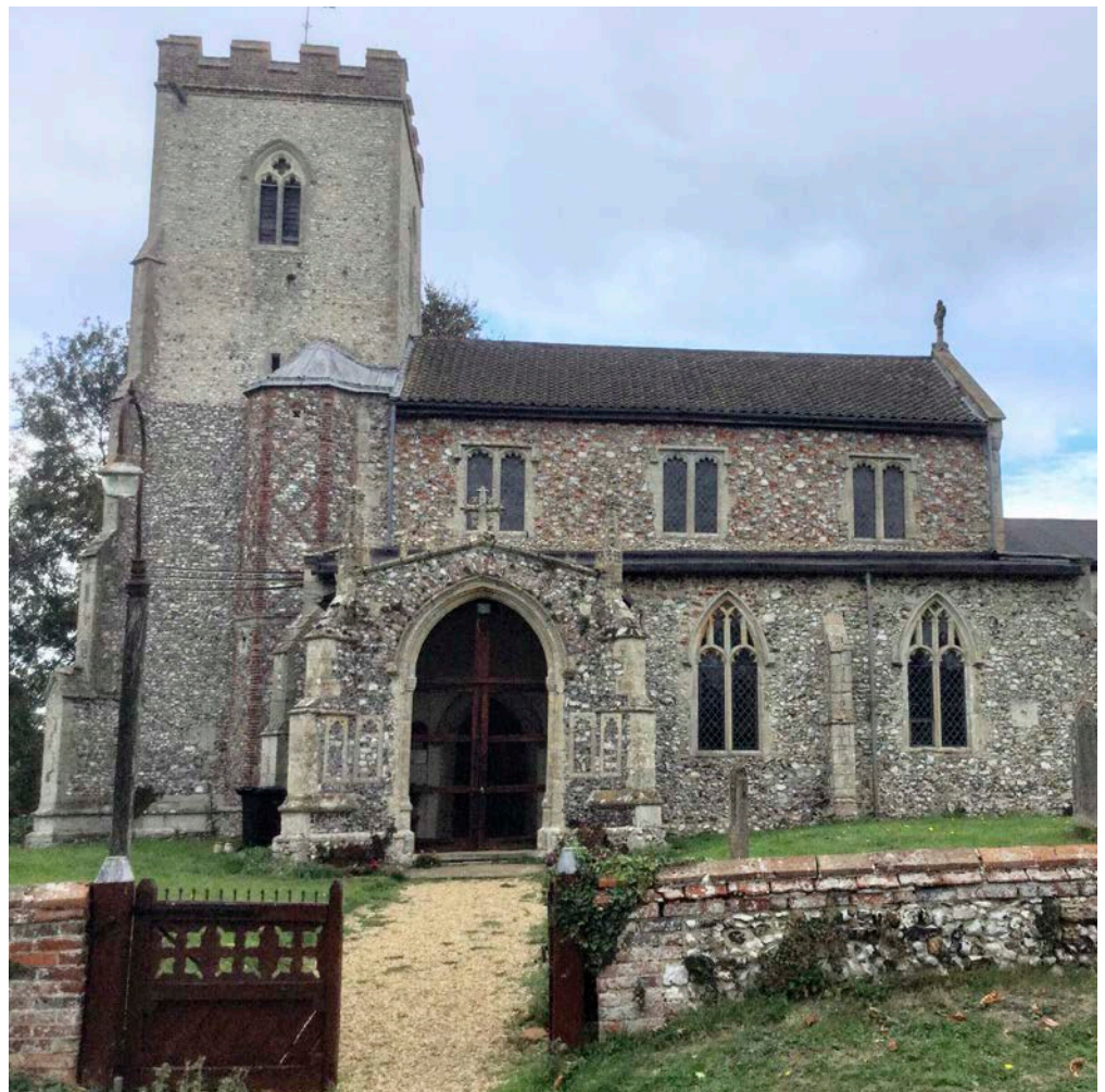
Figure 10: St Andrew's Church, Little Massingham. Flint and limestone rubble with Lincolnshire Limestone dressings. The clerestory is faced with Red Chalk, Lincolnshire Limestone and Quaternary Flint.
