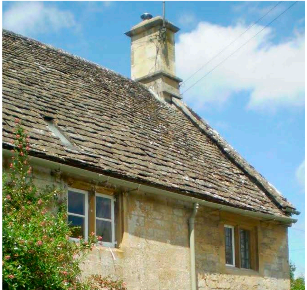
Figure 16: Cottage roof, Taynton. Cotswold Stone slate.
