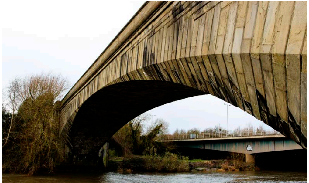
Figure 8: Over Bridge, near Gloucester. Pennant Sandstone.
