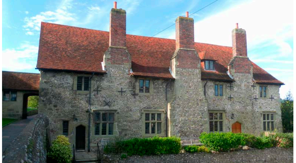
Figure 15: Parsonage, Eastbourne. Flint nodules and pebbles, with occasional blocks of ironstone and quoins of Eastbourne Sandstone.
