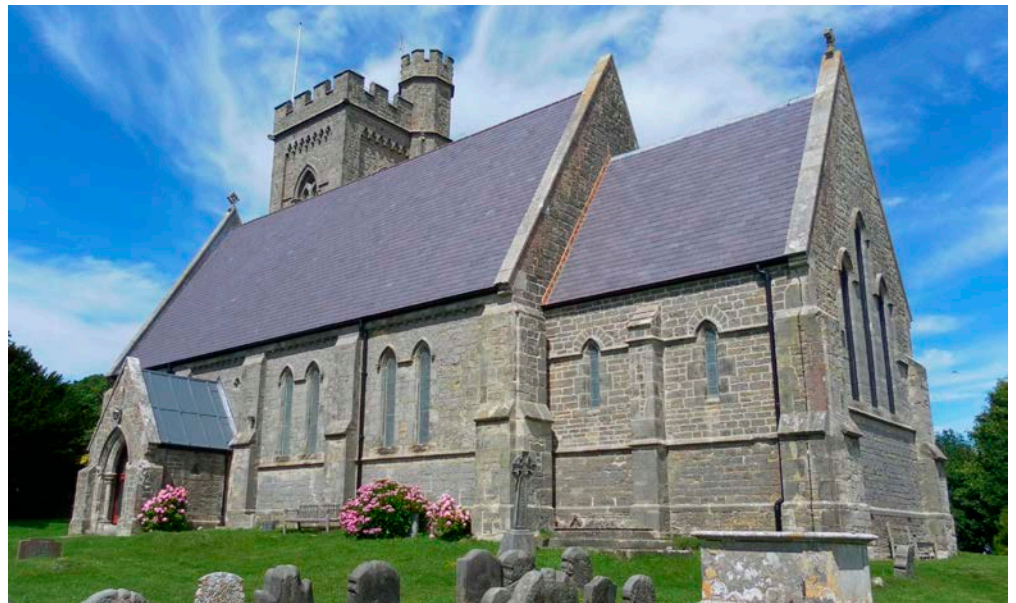
Figure 6: St Andrew's Church, Fairlight. Cliff End Sandstone.
