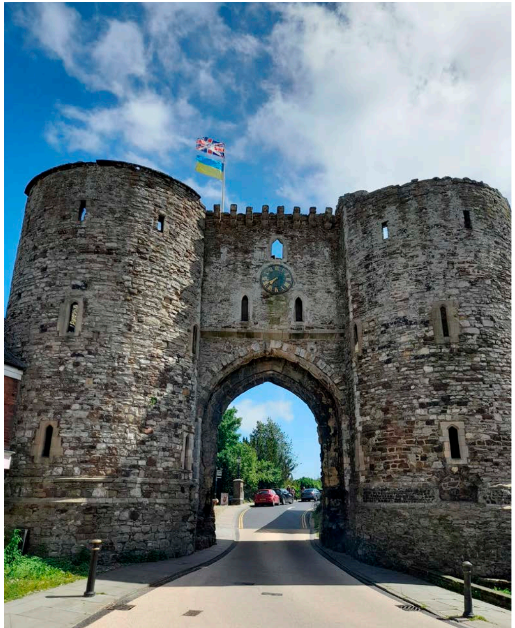
Figure 5: Landgate Arch, Rye. Rye Ironstone and Wealden Sandstone, including Ashdown Sandstone.
