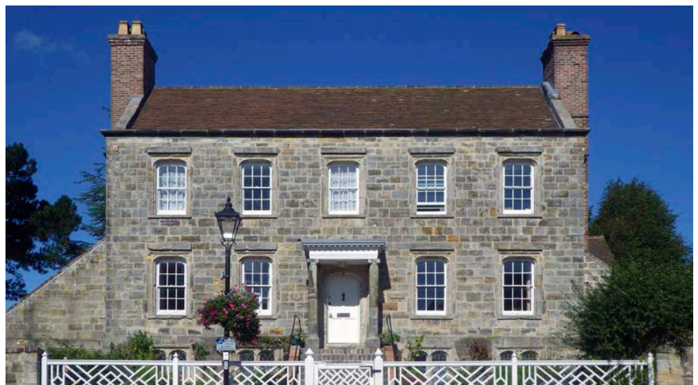
Figure 9: House, Main Street, Mayfield. Tunbridge Wells Sandstone with Ardingly Sandstone.
