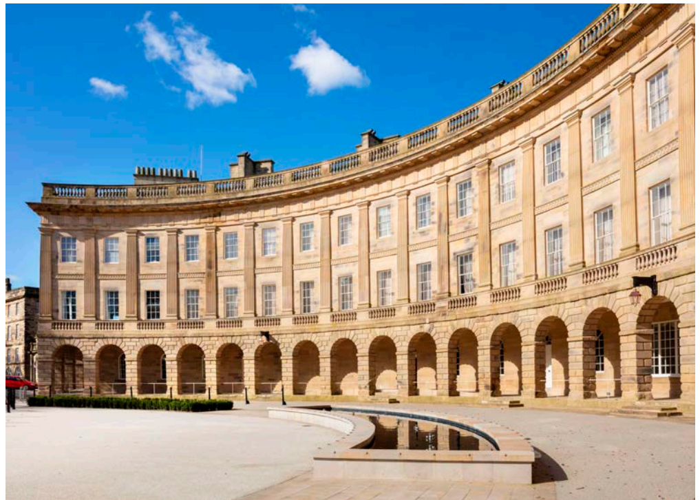
Figure 10: The Crescent, Buxton. Corbar Grit.
