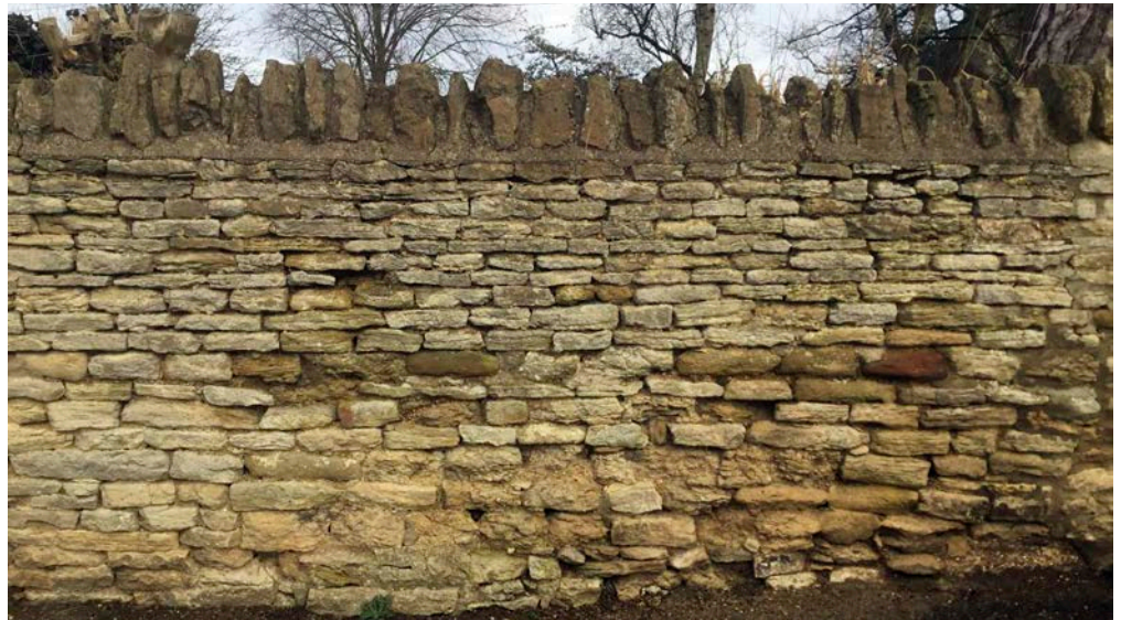
Figure 21: Churchyard wall, Ravenstone. Forest Marble and Cornbrash with Blisworth Limestone and ironstone.
