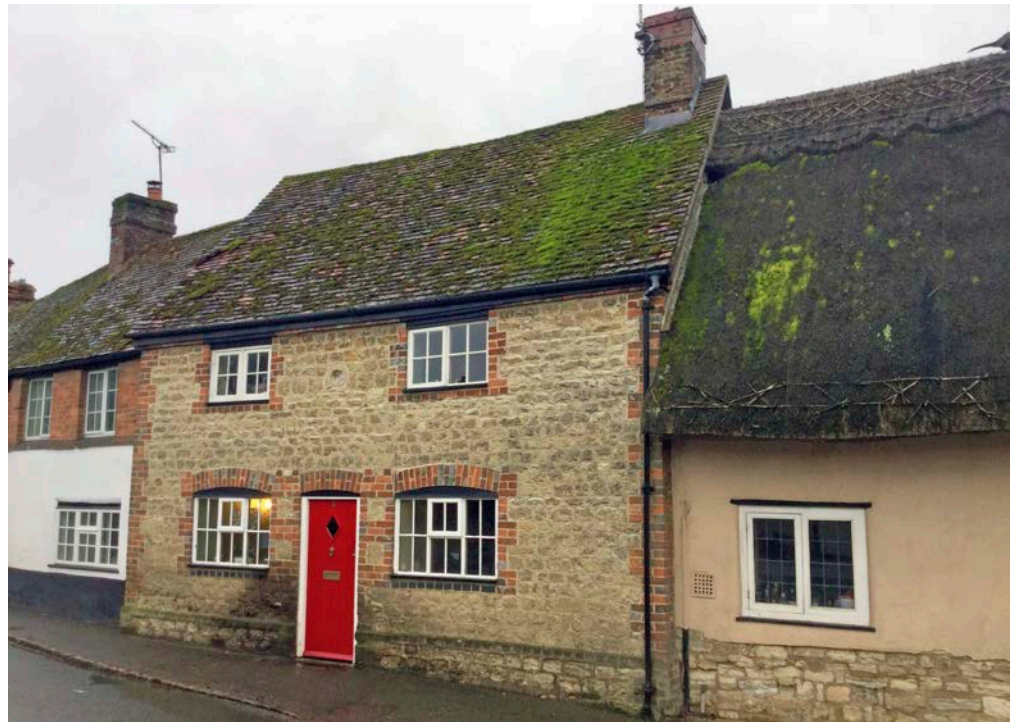
Figure 27: Cottages, Aylesbury Road, Cuddington. Portland Limestone (Buckinghamshire type) rubblestone.
