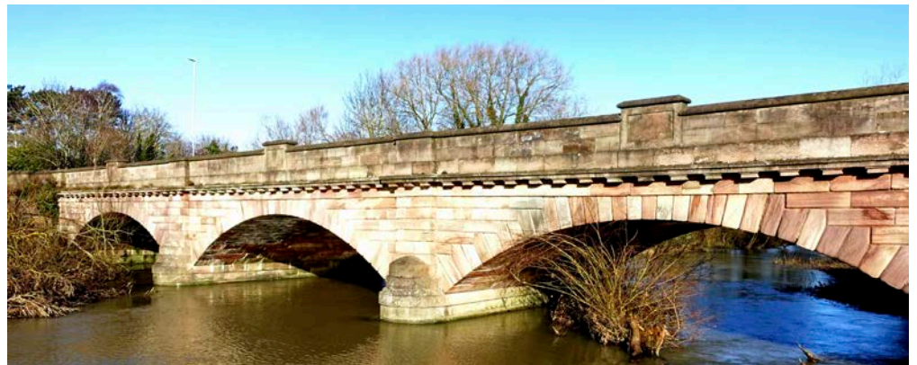
Figure 59: Stony Stratford Bridge over the River Ouse. Ashover Grit (Marsden Formation).
