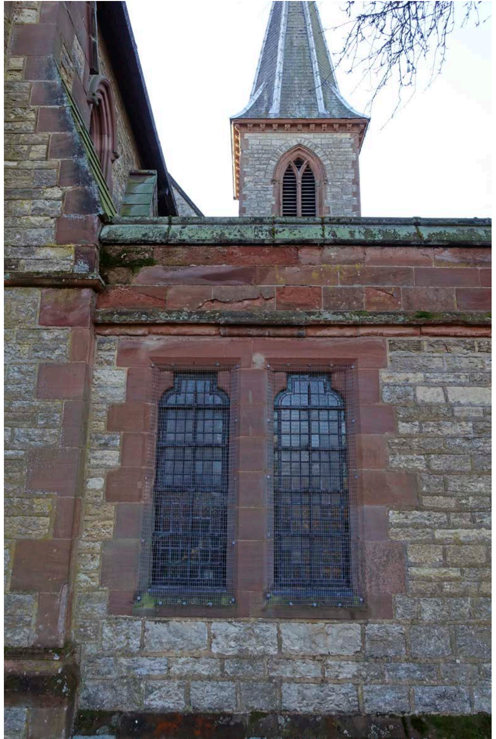
Figure 61: Church of St George the Martyr, Wolverton. Blisworth Limestone with Hollington Stone dressings.
