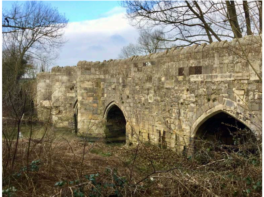
Figure 19: Thornborough Bridge, Thornborough. Blisworth Limestone.
