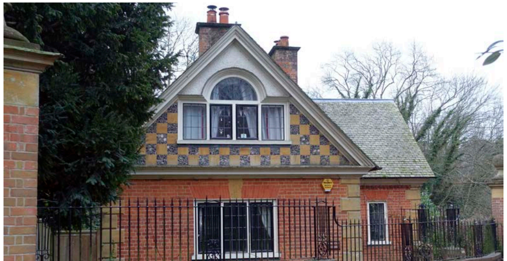
Figure 63: The Lodge Cottage, Henley Road, Medmenham. Brick with knapped flint and Ham Hill Stone chequerwork.
