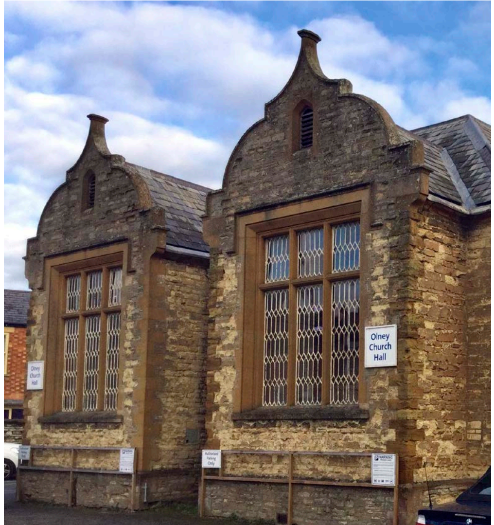
Figure 18: Olney Church Hall, Olney. Blisworth Limestone with Marlstone and weathered ironstone.
