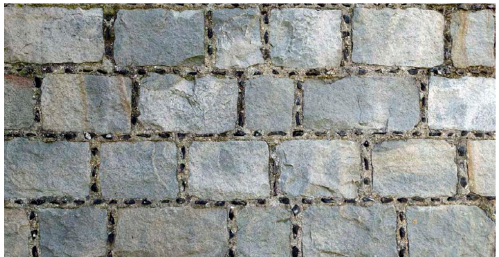
Figure 49: Detail of the walls of the Church of St Michael and All Angels, Halton. Sarsen stone blocks with flint galleting.
