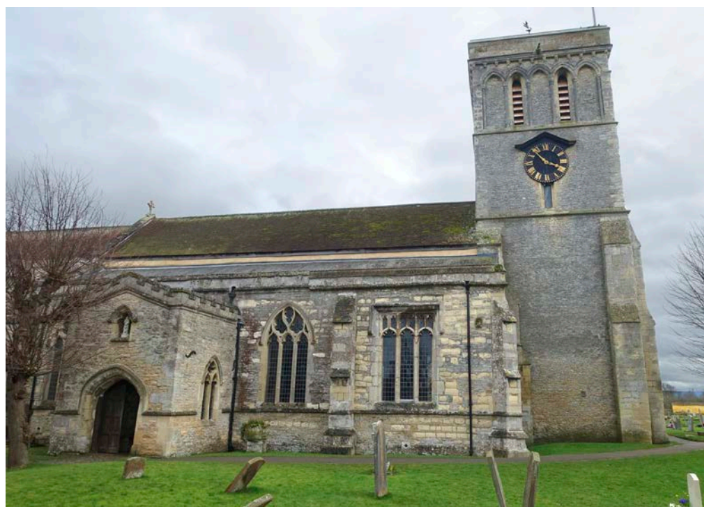
Figure 25: Church of St Mary the Virgin, Haddenham. Portland Limestone (Buckinghamshire type) and Purbeck Limestone (Buckinghamshire type).
