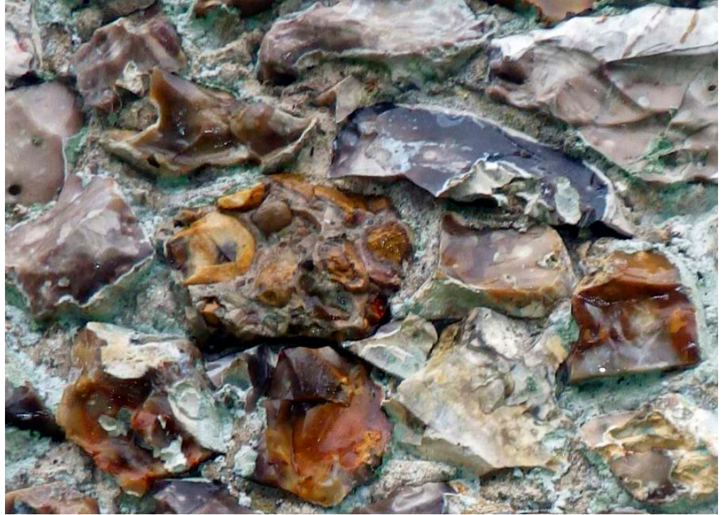
Figure 42: Church of St Botolph, Bradenham. Bradenham Puddingstone with Quaternary Flint nodules.
