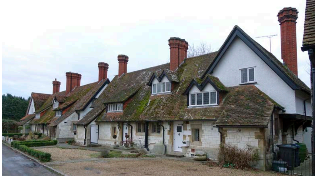
Figure 38: Cottages, Bockmer End, Medmenham. Chalk block.
