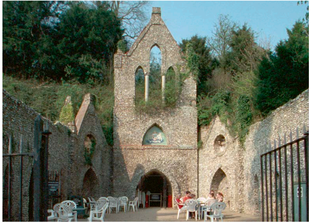
Figure 16: Hellfire Caves, West Wycombe. Flint rubble.
