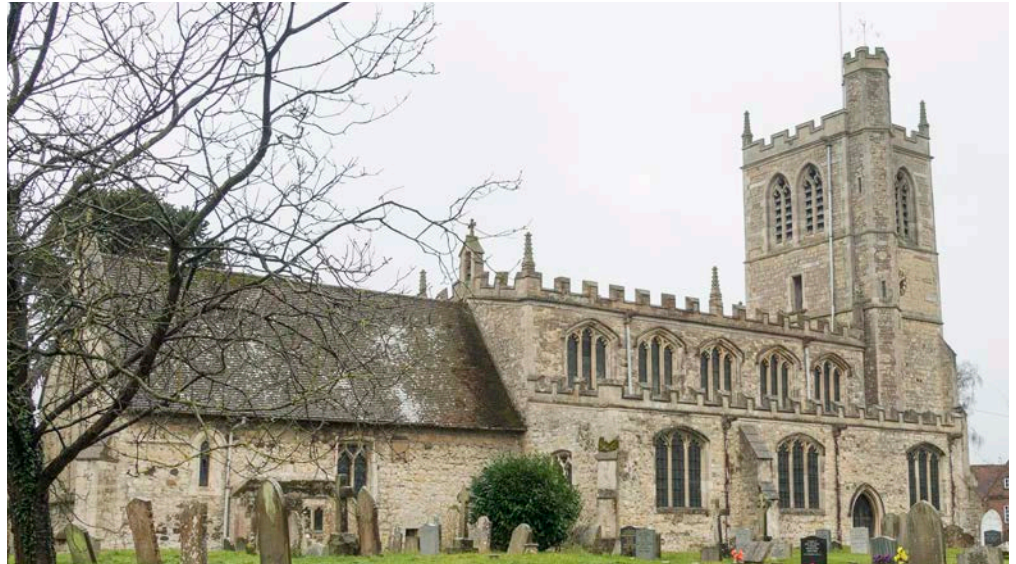
Figure 46: Church of St Peter and St Paul, Wingrave. Portland Stone (Buckinghamshire type), with False Puddingstone and glacial pebbles and cobbles.
