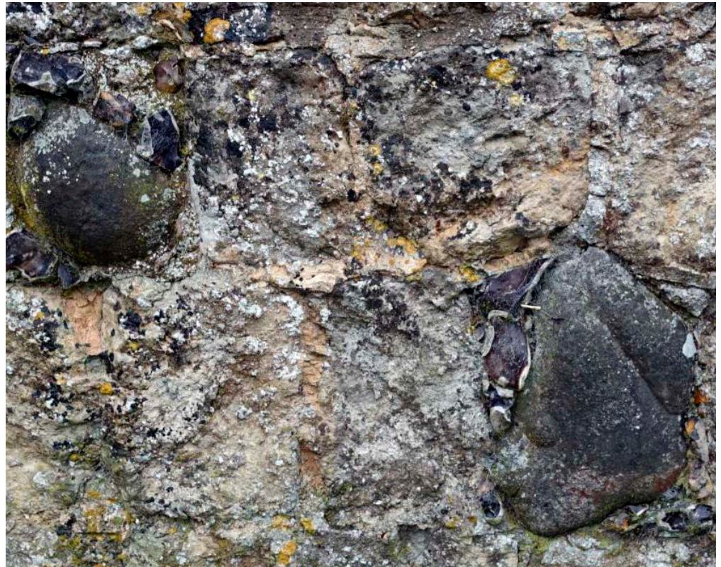
Figure 31: Roadside wall, Hartwell Park, Aylesbury. Bowel Stones in Portland Limestone (Buckinghamshire type).
