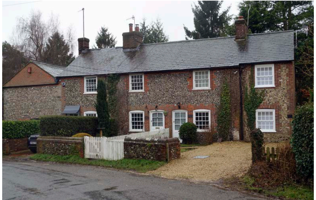
Figure 51: Cottages, Hughenden. Quaternary Flint nodules and Welsh Slate roofs.
