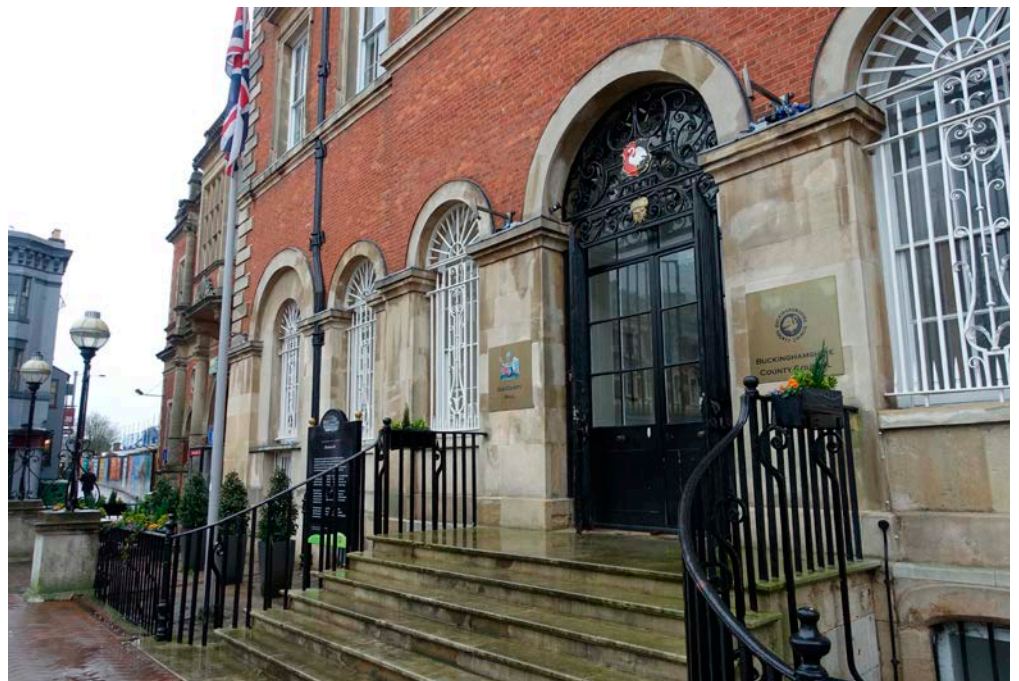
Figure 67: Old County Hall and Crown Court, Market Square, Aylesbury. Brick with Ketton Stone.
