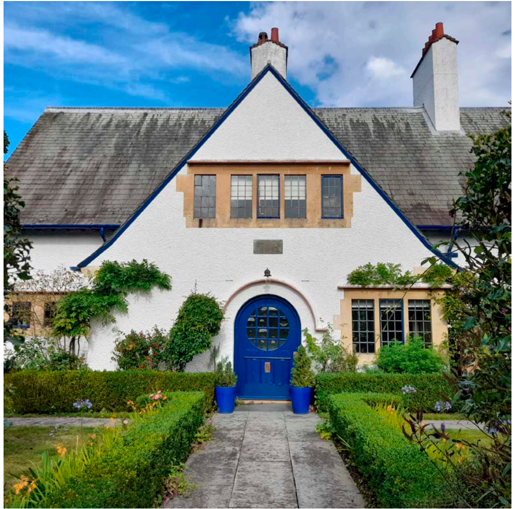
Figure 73: Holly Mount, Penn Road, Knotty Green. Bath Stone dressings and Cumberland Green Slate roof.
