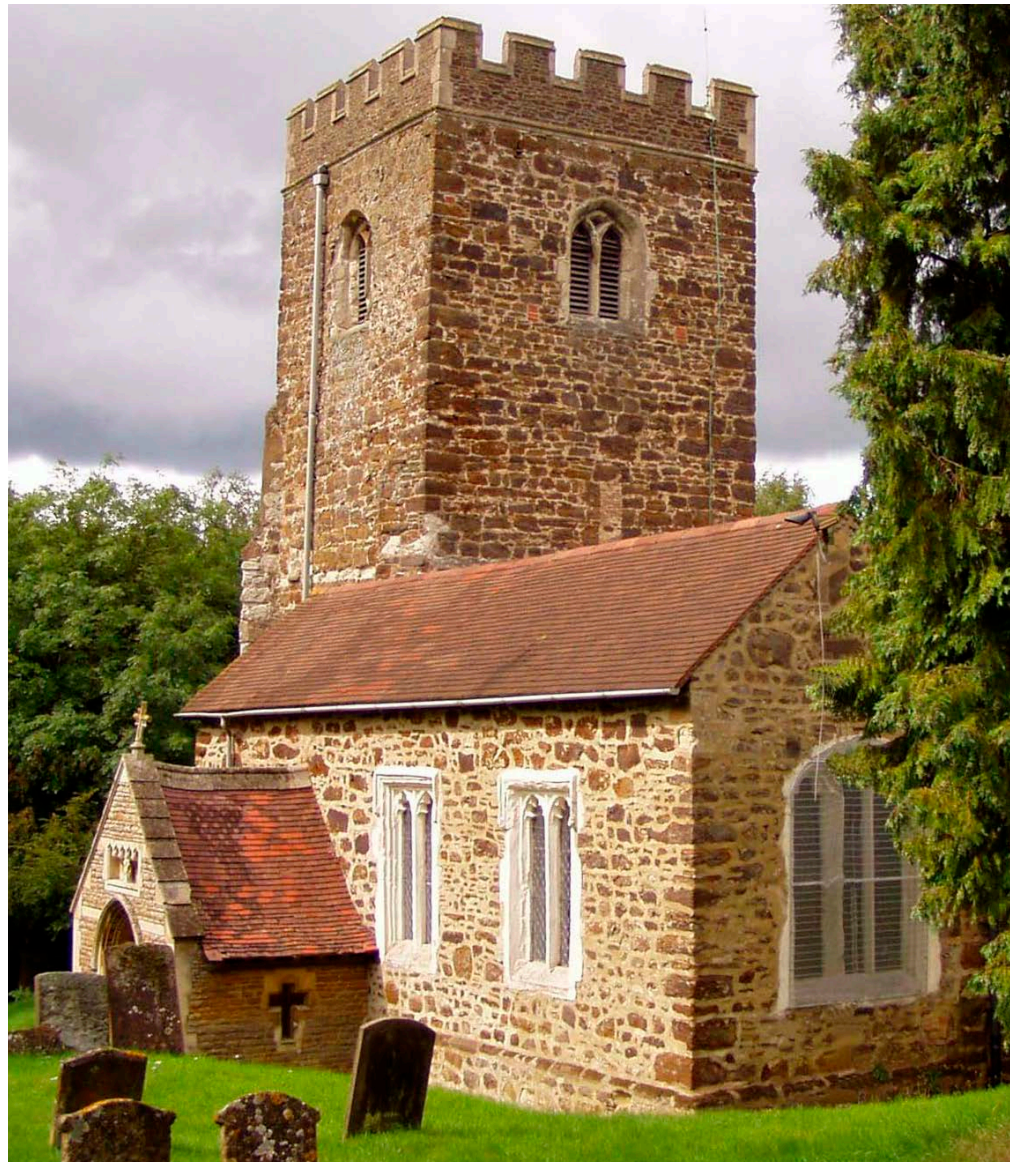
Figure 7: Church of All Saints, Bow Brickhill. Brickhill Ironstone with dressings of Totternhoe Stone and Middle Jurassic limestone.
