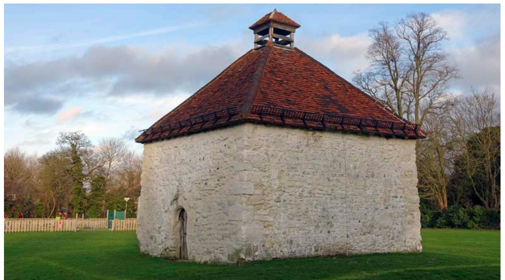
Figure 14: Dovecote, Monks Risborough. Chalk block and rubblestone.
