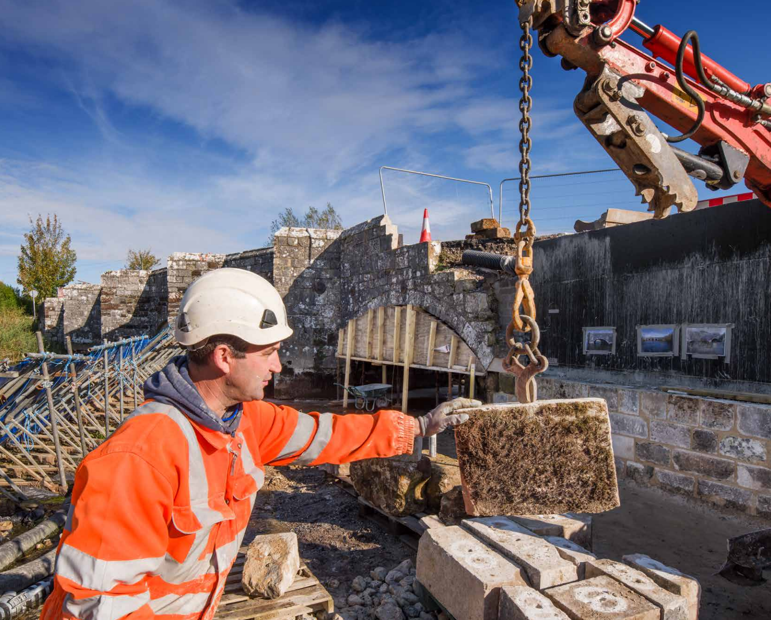
Construction workers on site at East Stoke, Dorset. © Historic England Archive
