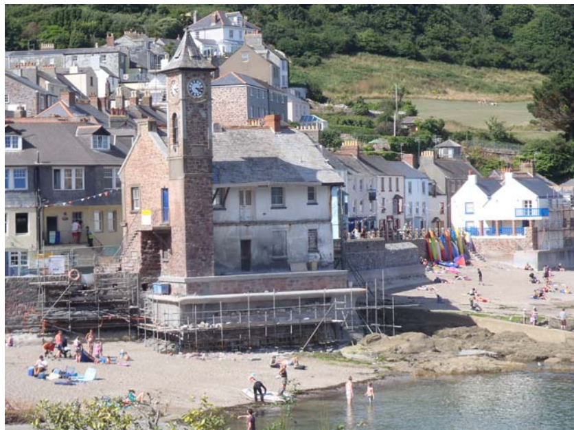
Repair work on the Kingsand Institute © John Grimes Partnership Ltd.
