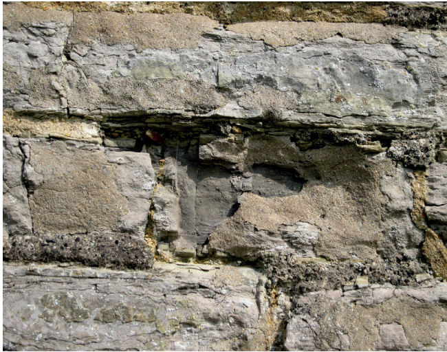
Consolidation of decaying Blue Lias stone was carried out using NHL 2 repair mortars 14 years ago. The mortar is still intact but it is not acting sacrificially, and the stone continues to decay. (Photo: Alison Henry)
