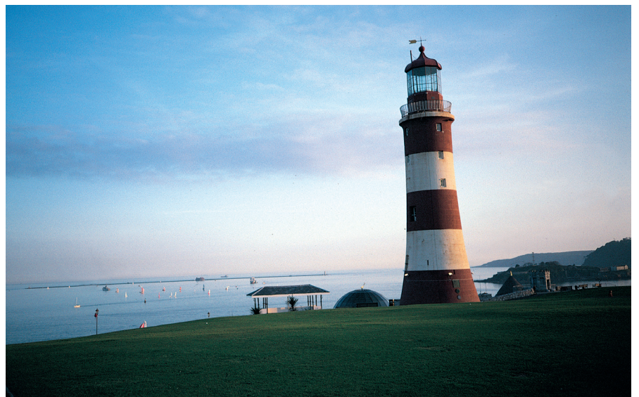
The remains of Smeaton’s Eddystone lighthouse today. John Smeaton carried out extensive research into hydraulic lime and pozzolans to inform his design of the third Eddystone Lighthouse (1756–1759), 12 miles south of Plymouth in Devon. He settled on Blue Lias lime mixed with Italian pozzolana. The lighthouse survived for over 120 years, and only had to be dismantled because the bedrock on which it was built was undermined by the sea, causing the tower to sway in strong seas. The upper part of it was reconstructed on Plymouth Hoe, but the lower part remains in situ, as it was found to be too strong to dismantle. (Photo: John Stewart)
