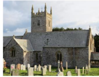
Southwest corner showing nave and transept roof abutment at 45°
