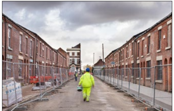
Regeneration of Victorian terraced housing in Toxteth, Liverpool
