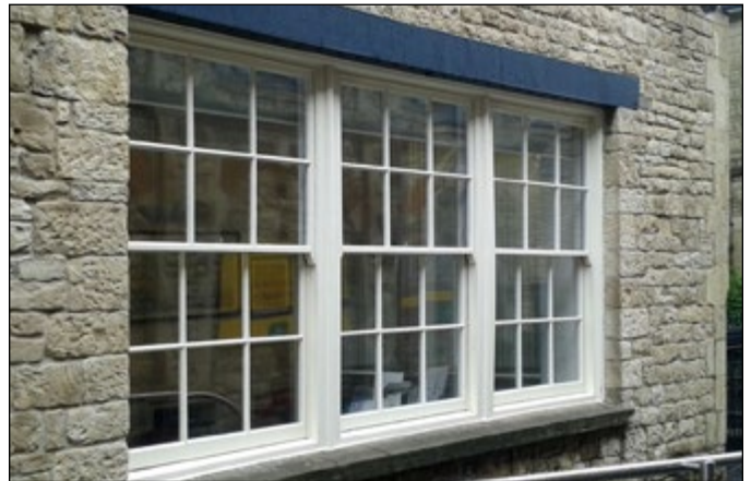
Timber sash windows, The Engine House, Swindon
