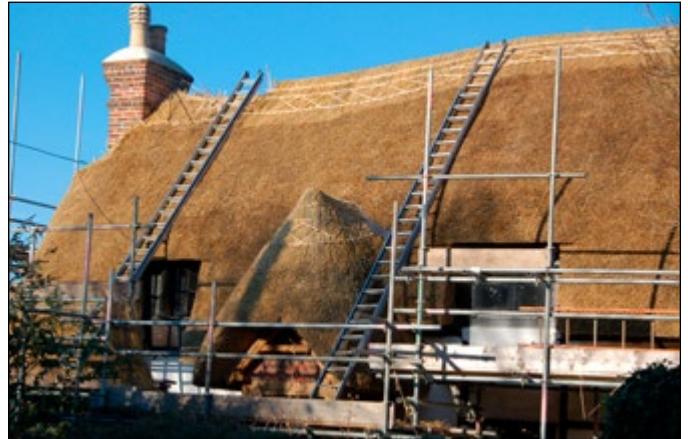
Re-thatching a cottage
