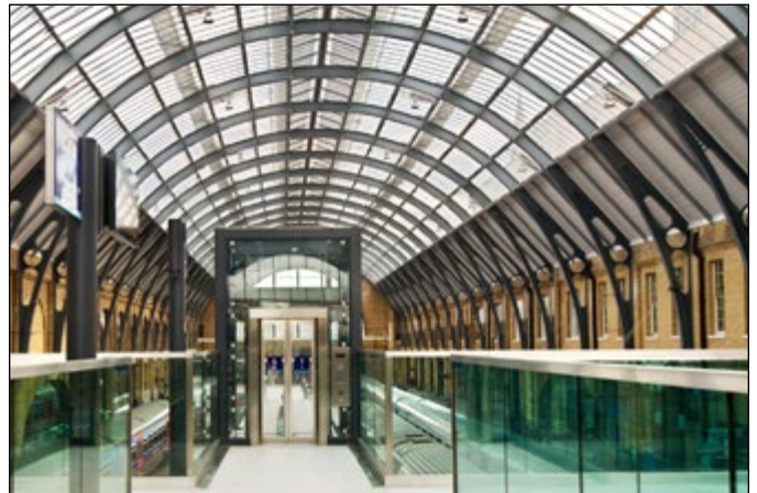
Photovoltaic cells installed in the glass roof above King's Cross Station, London
