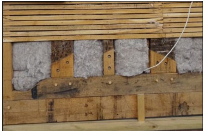
Insulation in timber-framed wall
