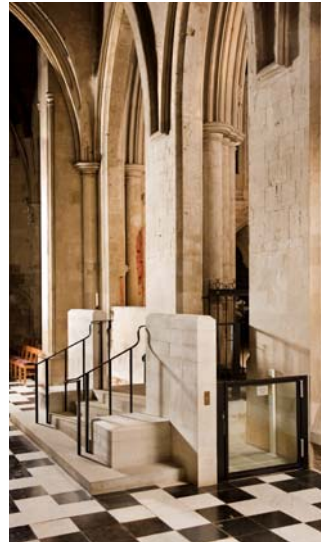
Top: stairway, with wheelchair lift on right
